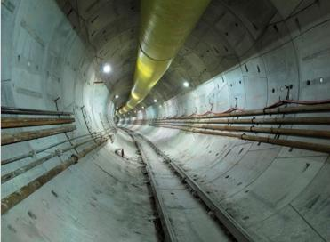
Figure 10.21 Precast Concrete Tunnel Lining
