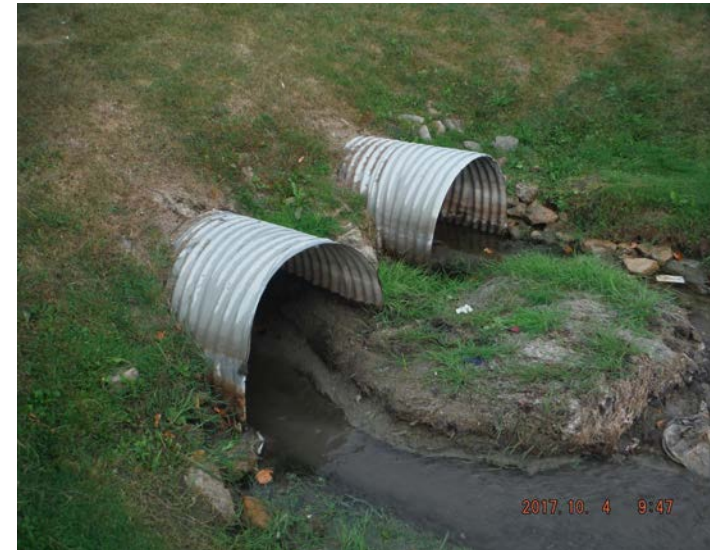
Photo 39: Downstream twin culvert inlet
