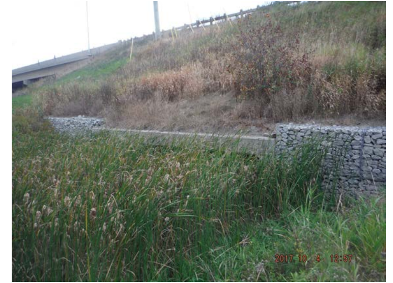
Photo 12: Facing culvert outlet at Langstaff Road
