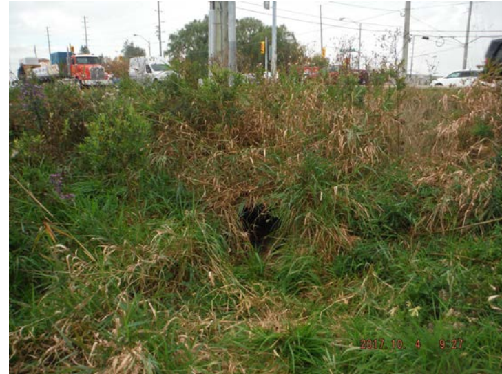
Photo 34: Facing culvert inlet
