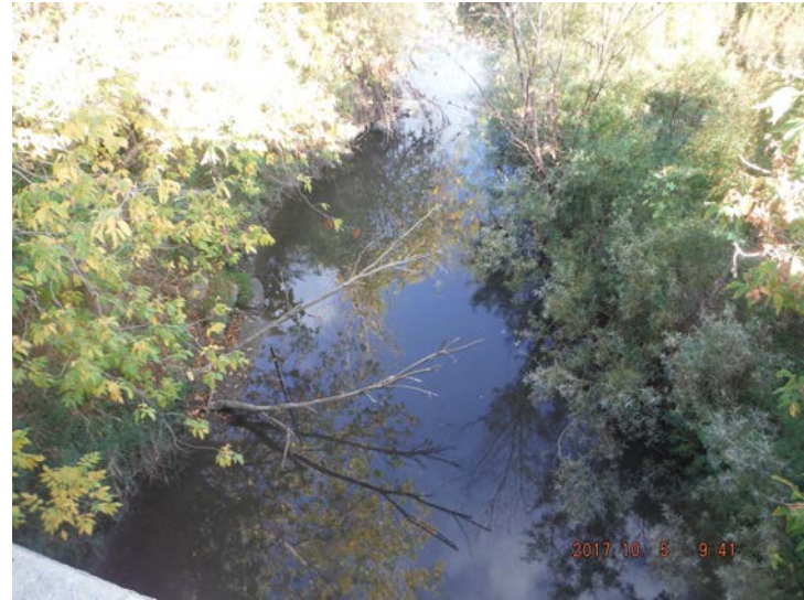
Photo 17: Overview facing upstream from the structure
