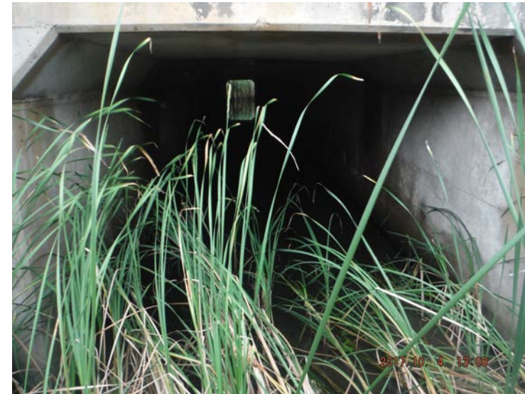
Photo 15: Looking through the culvert inlet at the off-ramp
