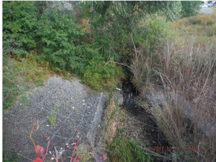
Photo 25: Overview facing upstream from the structure
