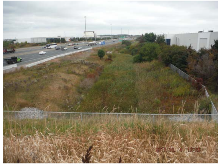
Photo 9: Overview of culvert inlet at Langstaff Road
