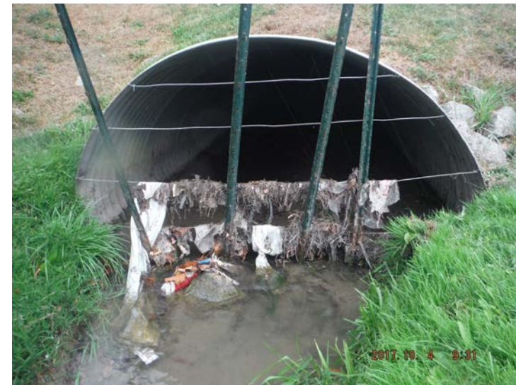
Photo 37: Facing downstream culvert outlet at Langstaff Road and Dufferin Street
