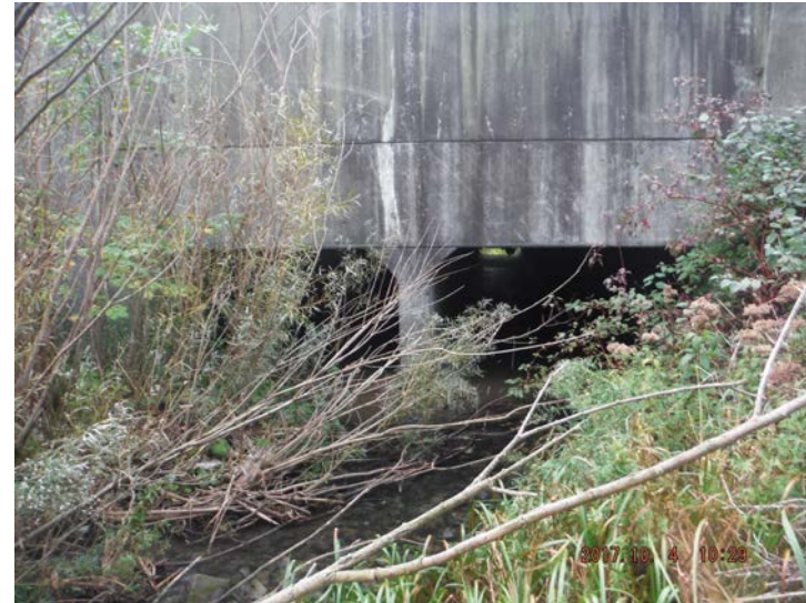
Photo 26: Downstream view facing the structure
