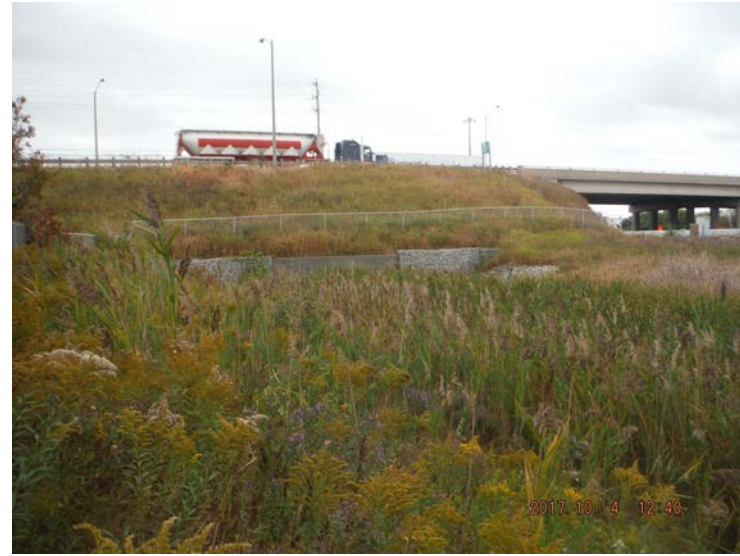
Photo 10: Facing culvert inlet at Langstaff Road
