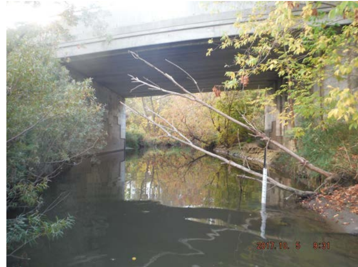
Photo 18: Downstream view facing the structure
