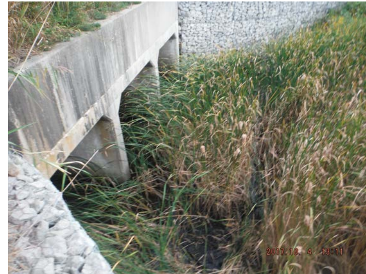
Photo 14: View of the culvert inlet at the off-ramp
