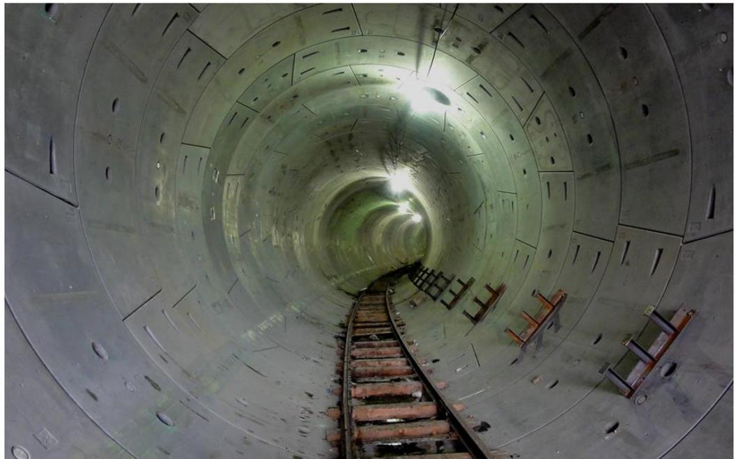
**Concrete Segmental Tunnel Lining**
