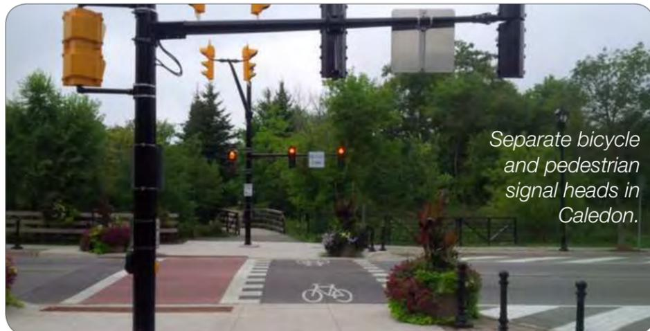
Separate bicycle and pedestrian signal heads in Caledon.
