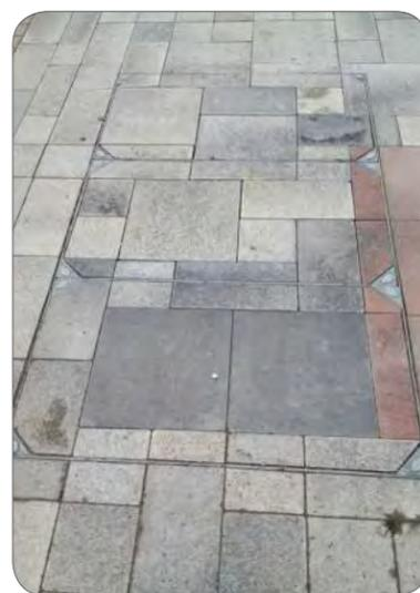
Image of recessed paver tray along the vivaNext corridor conceals utilities below in a paved area
