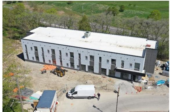
Site construction commenced the summer of 2021, in a manner to minimize disturbances and maintain safety for the clients and team who continue to actively use the other facilities on the site. This is the first time the Region has used modular, or prefabricated, construction for a housing development. Prefabricated construction uses components made off-site in a factory, which are then transported and assembled on-site to create a structure.
