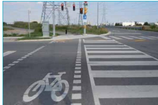
Figure 4.60- Mid-Block Signalized Cross-Ride of Flint Road North of Finch Avenue, City of Toronto
