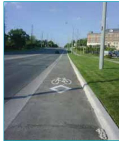
Figure 4.49 – Cycle Track along Stone Road in Guelph
