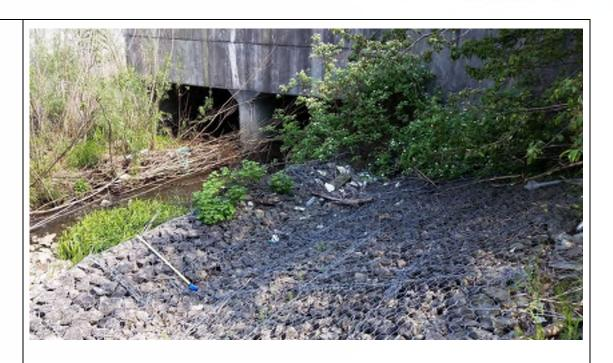
**Westminster Creek:** The Langstaff Road crossing consisted of a double-cell concrete box culvert. The gabion baskets near the crossing were in good condition.
