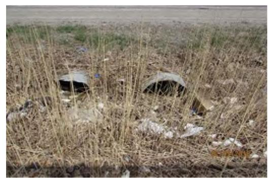
Photo 9: Existing Drainage Culvert Twin CSP 900 mm near St. 7+060, Downstream view
