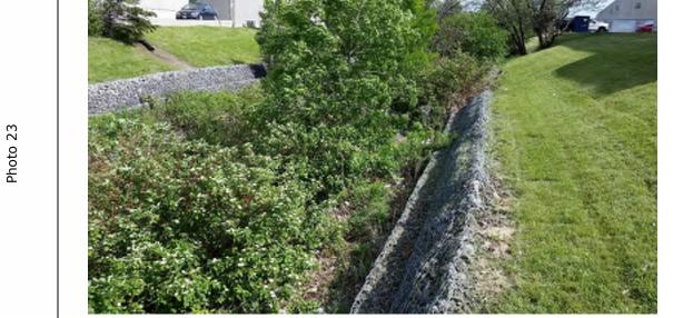
**Westminster Creek:** The channel corridor was armoured with gabion basket. The corridor was constrained between commercial lots.
