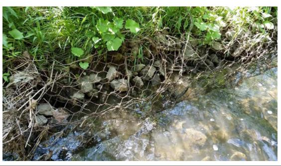
**Westminster Creek:** Some sections of the gabion basket wire meshing were eroded and missing stone.
