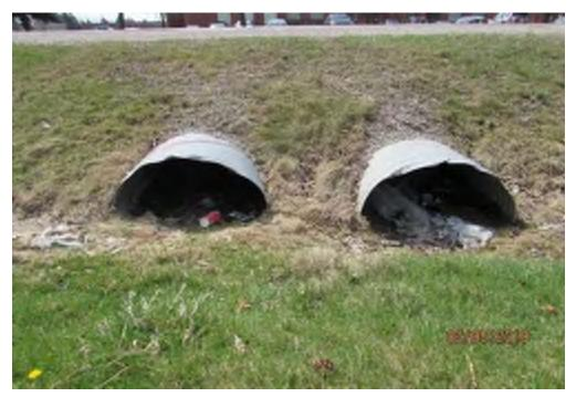
Photo 10: Existing Drainage Culvert Twin CSP 900 mm near St. 7+060, Upstream view
