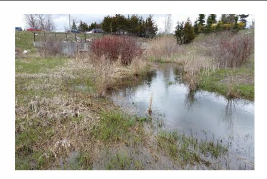
**Black Creek:** The realigned channel design followed a sinuous planform. Flow conditions were at bankfull capacity during the time of assessment due to recent rainfall.
