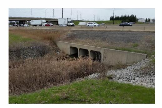
**Black Creek:** The channel formed into a wide vegetated swale near the Highway 400 crossing. The channel had been previously realigned and reinforced with riprap.
