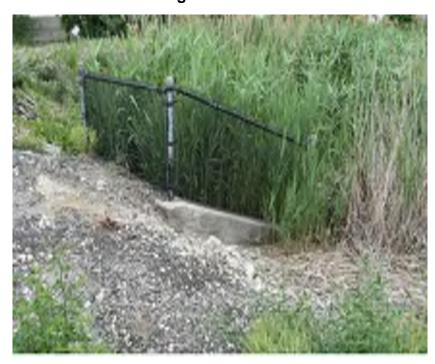
Photo 17: Outlet of 1650 mm diameter storm Sewer that crosses Langstaff Road and discharges to a ditch downstream of Langstaff Road in CN Property (Inlet Channel to Existing SWM Pond C)
