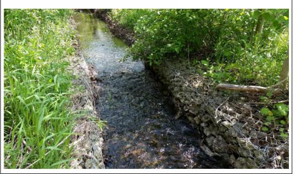
**Westminster Creek:** Upstream of the Langstaff Road crossing the channel and valley corridor were armoured with gabion basket. The channel was straight.
