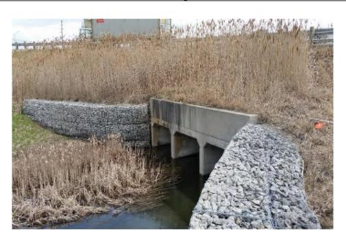
**Black Creek:** A triple-cell concrete box culvert was observed at the highway interchange crossing, south of Langstaff Road.
