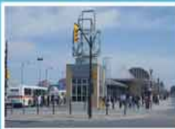
Transit Terminal Expansion
