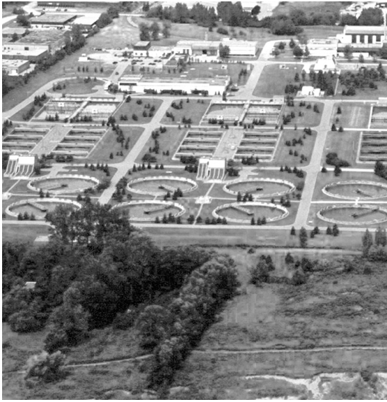
The York Durham Sewer System is state-of-the-art
