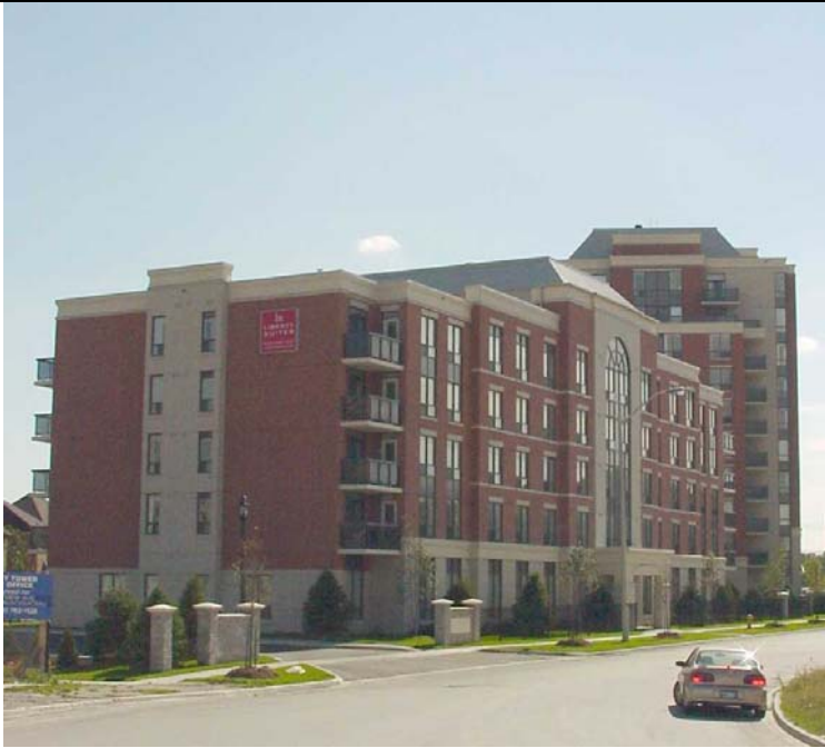
View – looking south on Times Avenue from Highway 7
