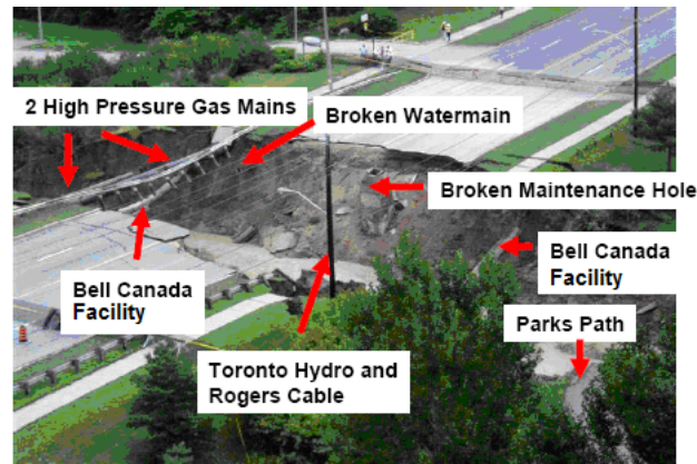
Finch Avenue Collapse
