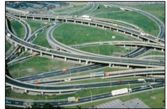
Roads that can withstand higher temperatures
