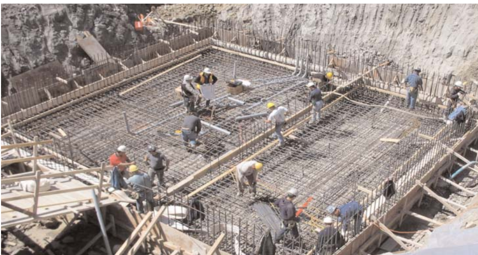
The Regional pumping station in King City is under construction
