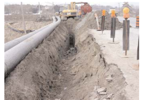
Entrance site for pipe-pull operation
