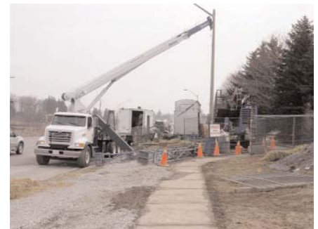
Directional drilling eastbound at Warren Road
