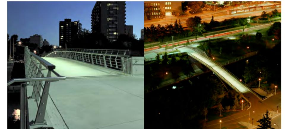
**Figure 121:** Cork Town Pedestrian Bridge: Soft light floods the bridge floor from glare free LED lighting in the handrail, allowing safe use of the bridge without trespass to the low light level landscape below.
