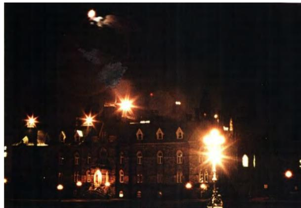
**Figure 119:** West Block, Parliament Hill: Glare vs. Visibility - Roof mounted security lights caused glare, obscuring view of the building and impairing security
