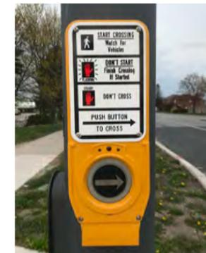
**Figure 212:** Audible Pedestrian Signals Are Important for Accessible Streets
