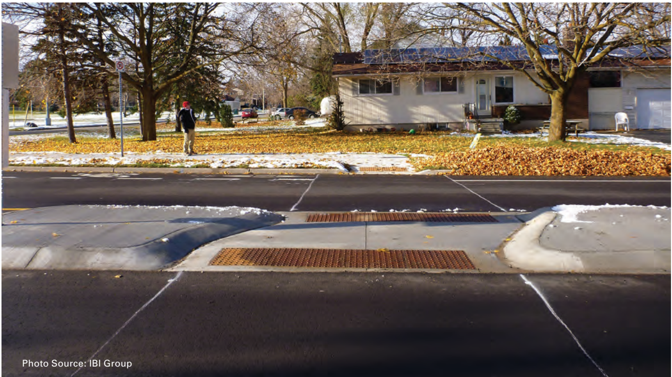
Exhibit 5-45. Use of detectable curbs to guide pedestrians through median refuge island
