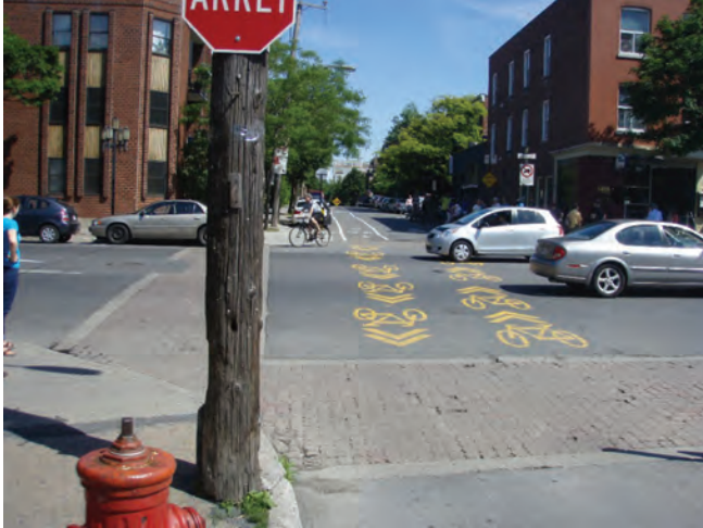
Pavement markings highlight cyclist path across an unsignalized intersection
