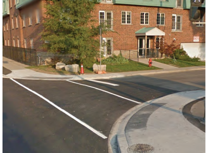
Crossings at unsignalized intersections must include curb ramps or depressions with tactile walking surface indicators
