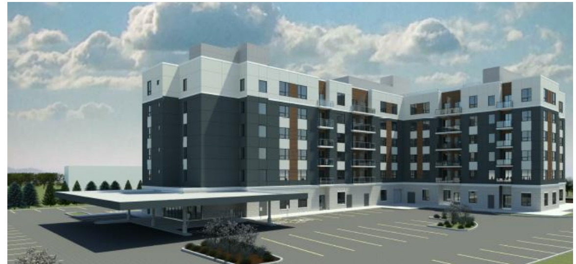
North-West view from Metro
