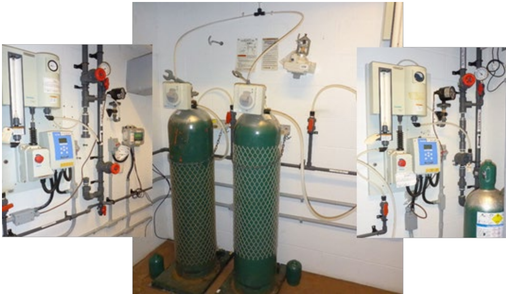
Figure 2-4. Well 3 Treatment Facility Chlorine Gas Feed Systems
