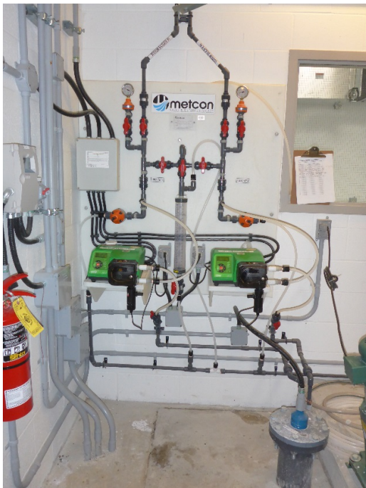
Figure 2-4. Well 3 Treatment Facility Chlorine Gas Feed Systems
