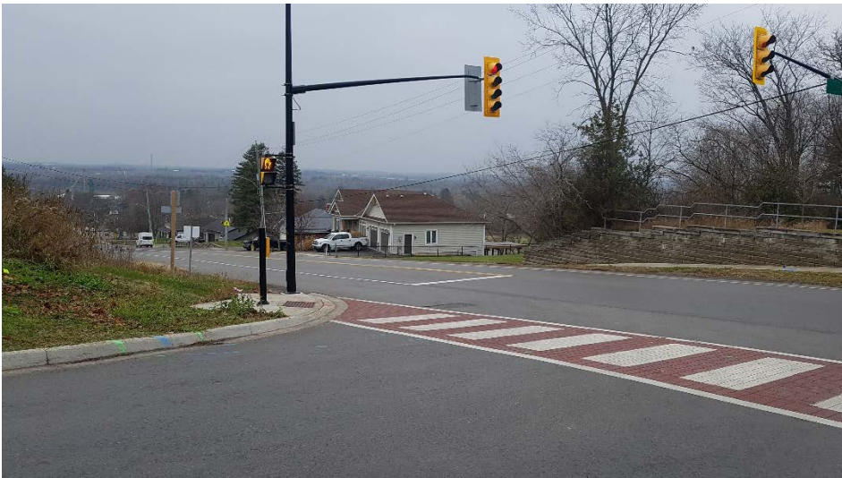
Image 25: View of disturbances associated with previous roadway improvements – asphalt roadway, concrete curbs and sidewalks, buried utilities.
