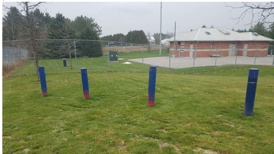
Image 20: View of area subjected to previous grading and construction activities associated with the installation of the well site.
