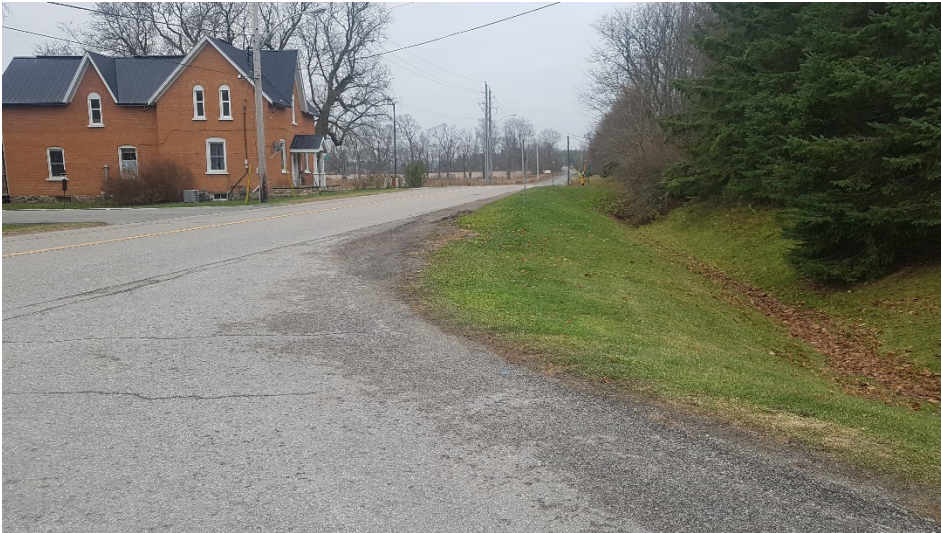
Image 9: View of disturbances associated with the asphalt roadways, gravel shoulders, deep drainage ditching, culverts and a residential structure.
