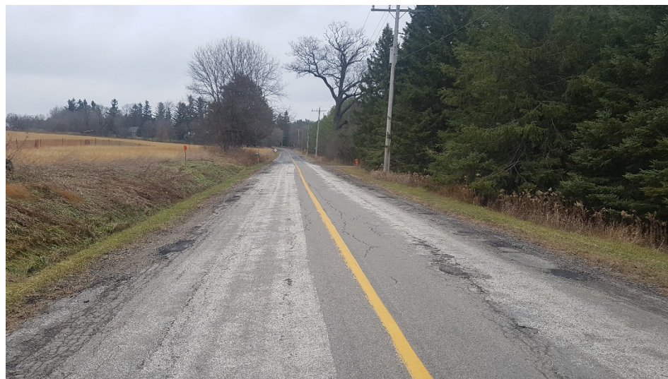
Image 18: View of disturbances associated with the asphalt roadway. Note the cut and embankment of the road bed within the surrounding slightly sloping terrain. Lands beyond the disturbed road ROW retain archaeological potential.
