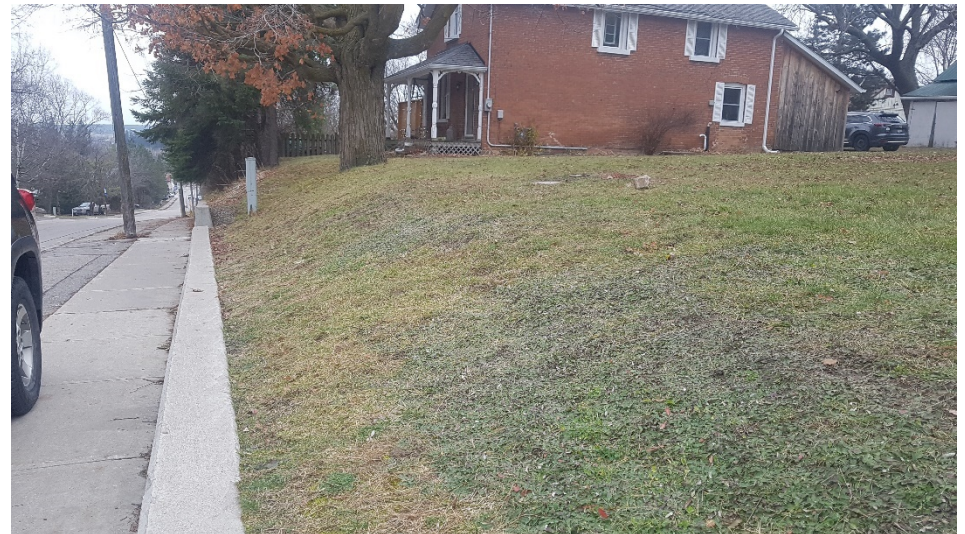
Image 4: View of disturbances associated with a cut slope, concrete sidewalk and barrier, and existing structures adjacent to the Mount Albert Wesleyan Methodist Pioneer Cemetery property limits.
