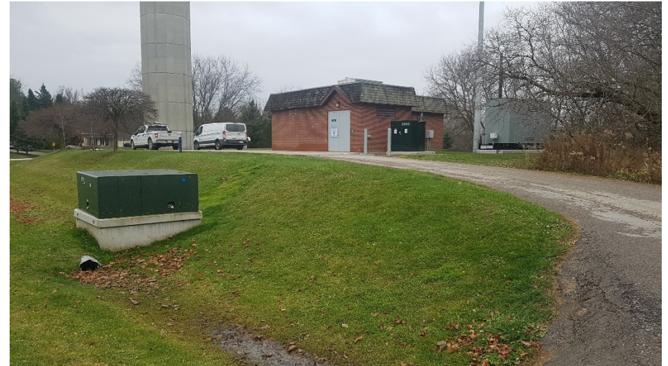
Image 6: View of disturbances associated with deep drainage ditching, an asphalt driveway and regional infrastructure (Mount Albert wells 1 and 2 and elevated tank).
