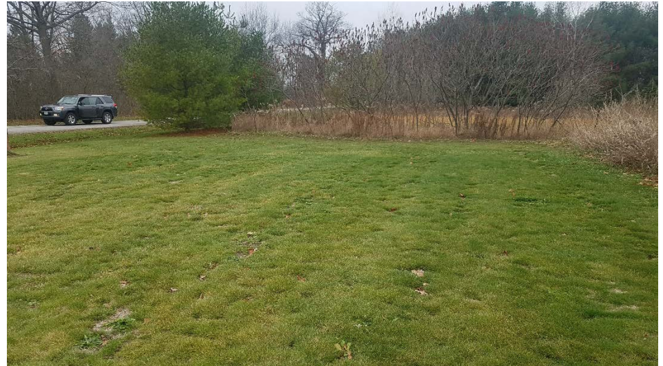
Image 22: View of area subjected to previous grading and construction activities associated with the installation of the well site.
