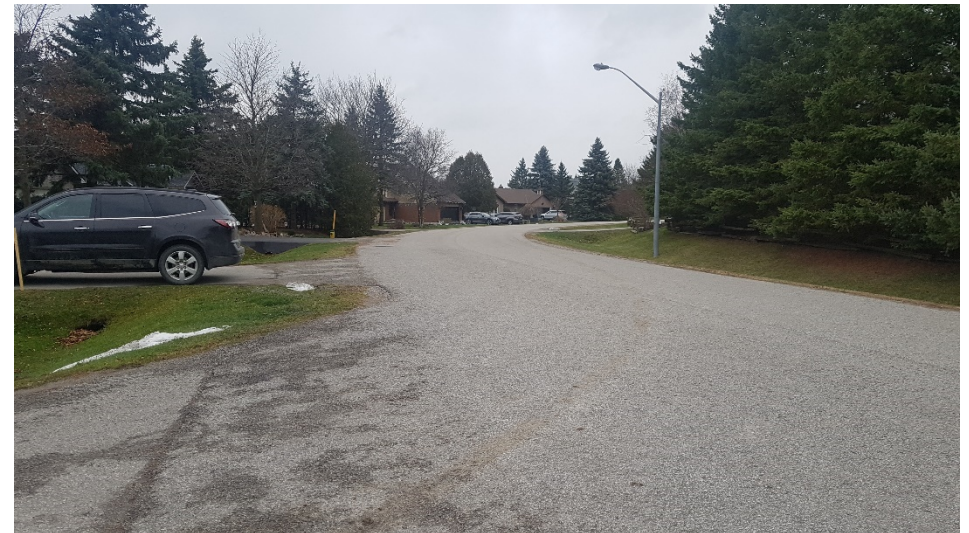
Image 8: View of disturbances associated with an asphalt roadway, intersecting driveways, deep drainage ditching, culverts, and residential structures.
