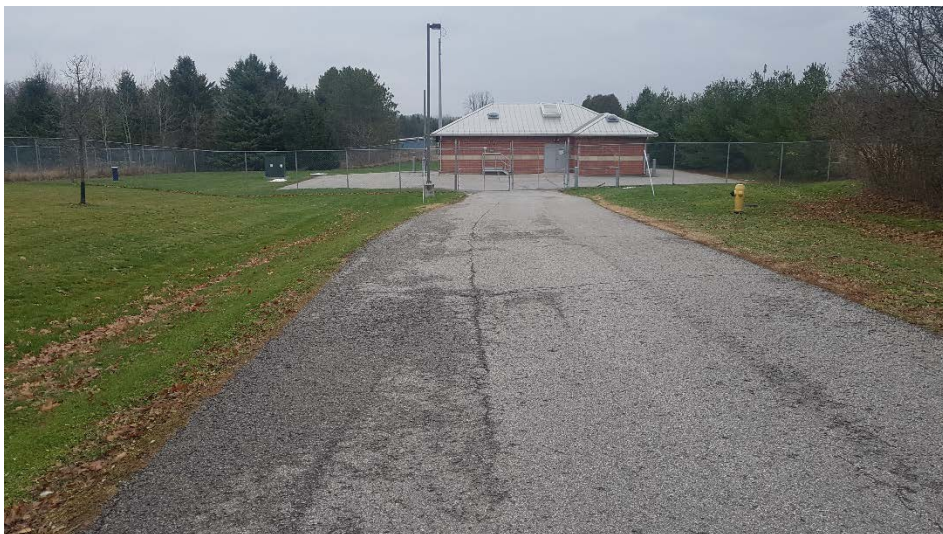
Image 19: View of disturbances associated with regional infrastructure (well 3).
