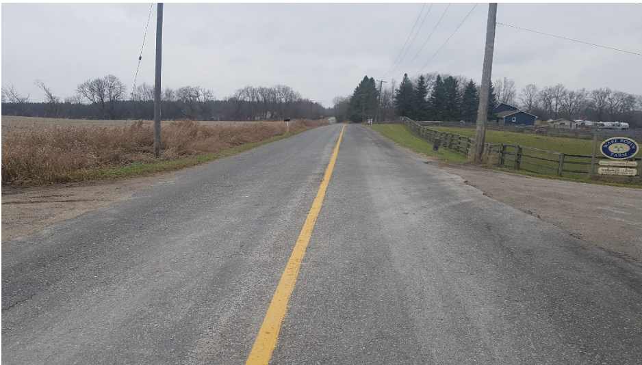
Image 13: View of disturbances associated with the asphalt roadway, intersecting gravel driveways and extant structures. Lands beyond the disturbed road ROW retain archaeological potential.
