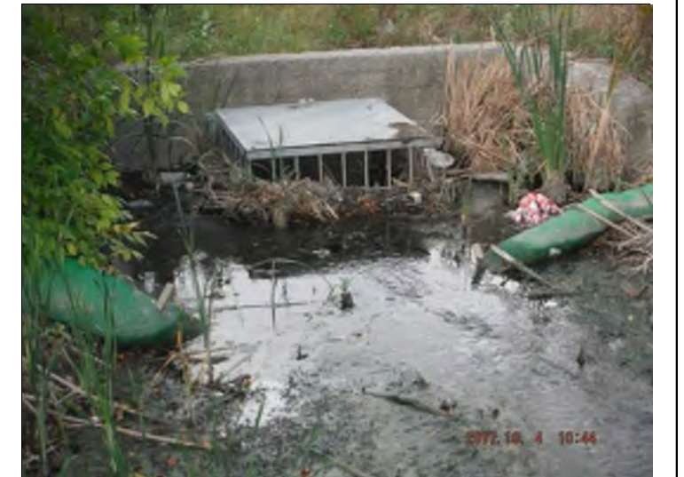
Photo 40: Downstream vertical culvert acting as a permanent barrier to fish passage upstream
