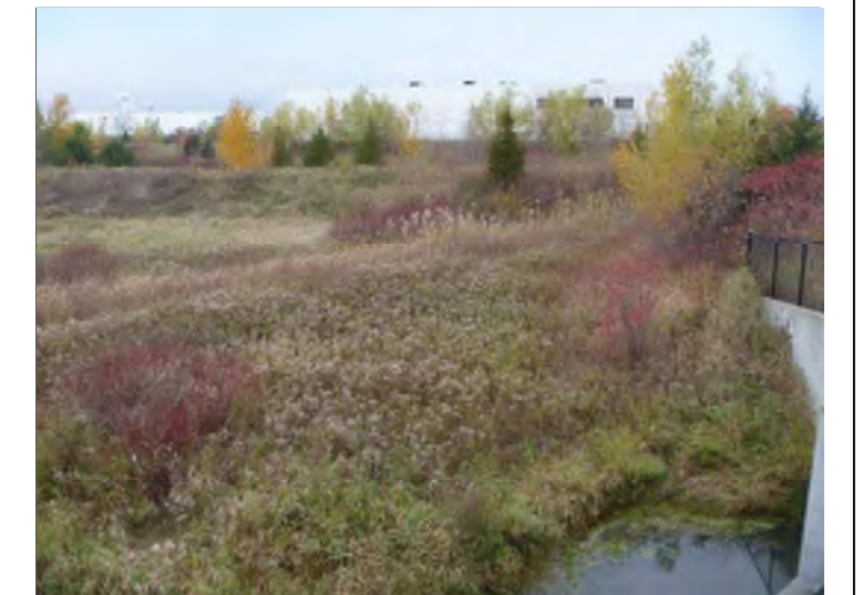
Photo 8: Overview facing upstream from the culvert inlet at Highway 400
