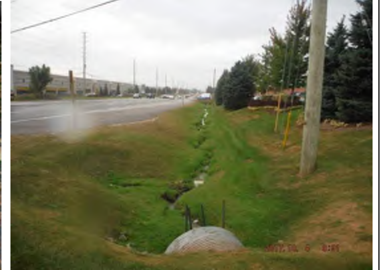
Photo 36: Downstream overview at Langstaff Road and Dufferin Street
