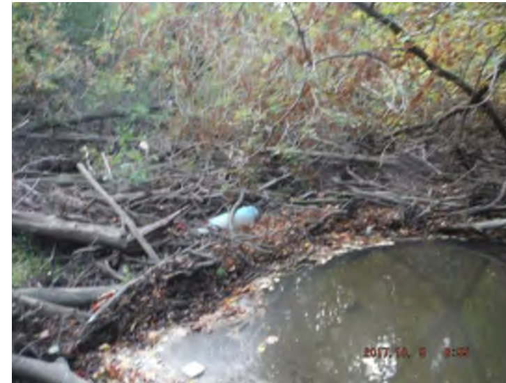
Photo 23: Downstream woody barrier
