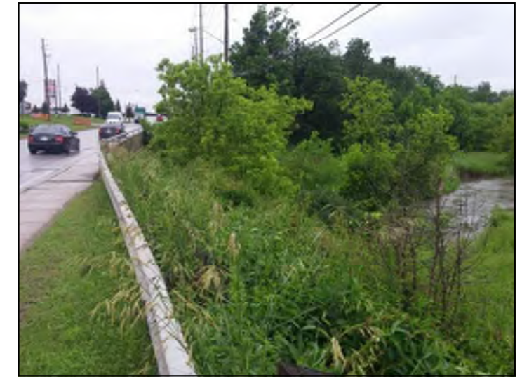
Photo 4: View of Unit 5 and Langstaff Road looking west, June 23, 2017.
