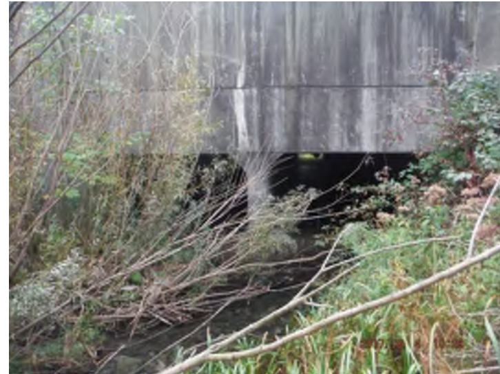
Photo 26: Downstream view facing the structure
