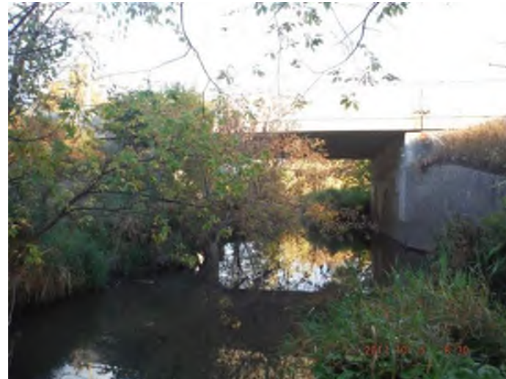
Photo 22: Upstream view facing the structure
