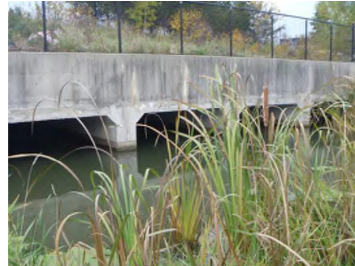
Photo 3: Facing the culvert outlet at Creditview Road
