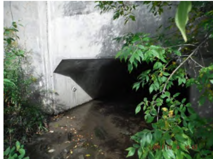
Photo 30: Upstream view facing the structure
