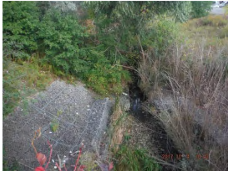
Photo 25: Overview facing upstream from the structure
