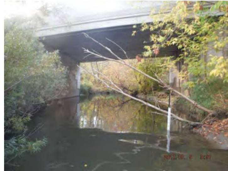
Photo 18: Downstream view facing the structure
