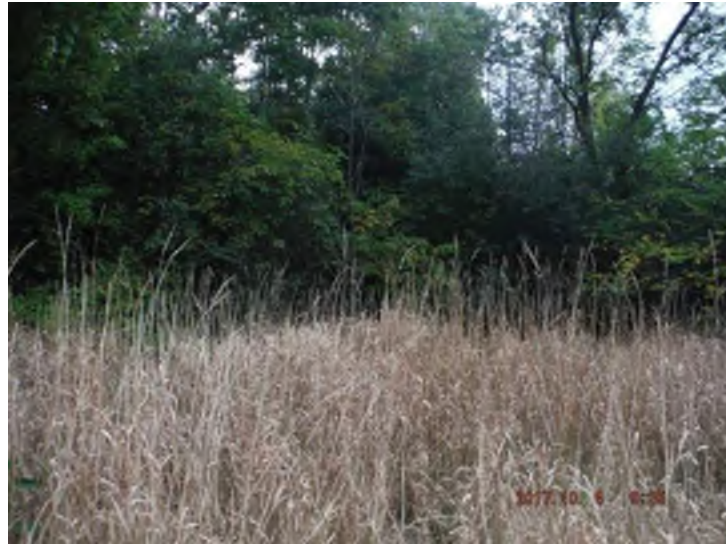
Photo 33: Overview facing upstream from the culvert inlet at Langstaff Road and Dufferin Street
