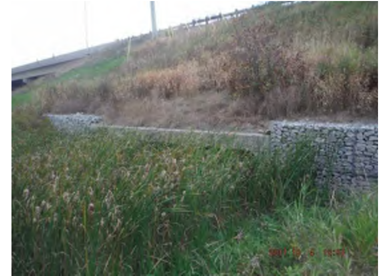
Photo 12: Facing culvert outlet at Langstaff Road
