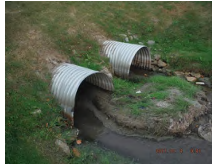
Photo 39: Downstream twin culvert inlet
