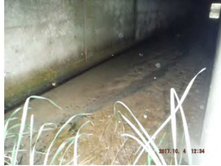
Photo 11: Looking downstream through the Langstaff Road culvert inlet
