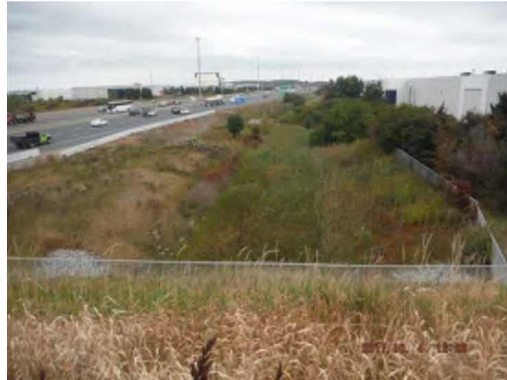
Photo 9: Overview of culvert inlet at Langstaff Road
