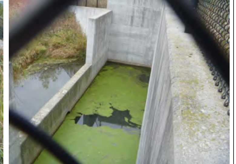
Photo 4: View of the overflow structure near the inlet at Creditview Road
