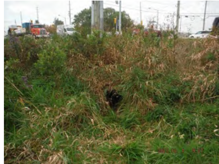
Photo 34: Facing culvert inlet
