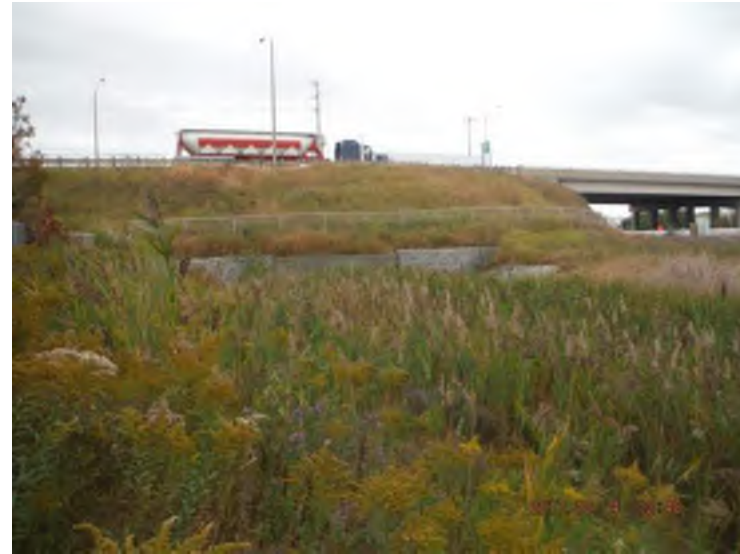
Photo 10: Facing culvert inlet at Langstaff Road
