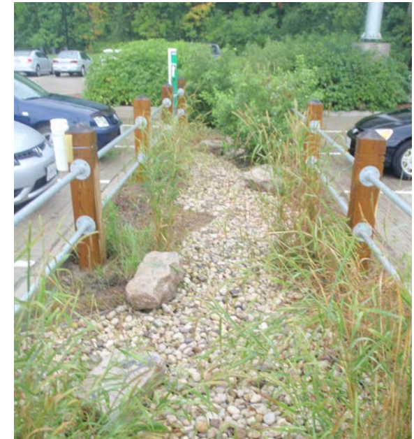
Bioretention cell incorporated into parking lot Source: Toronto Region Conservation Authority
