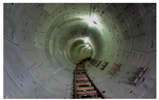
**Concrete Segmental Tunnel Lining**
