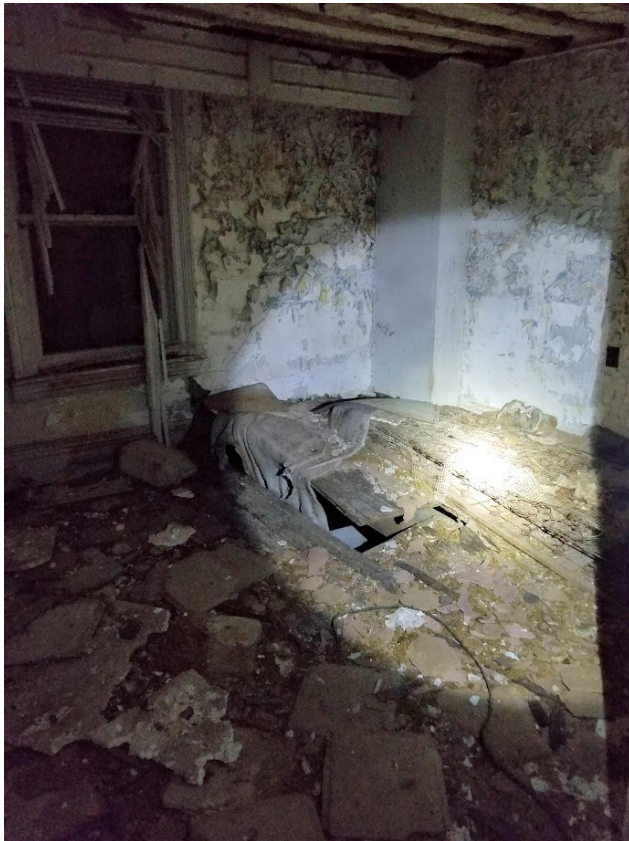
Deterioration of floor assembly
