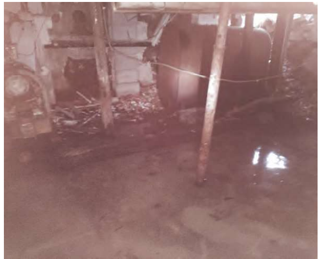
Furnace detail, crooked pipe support
