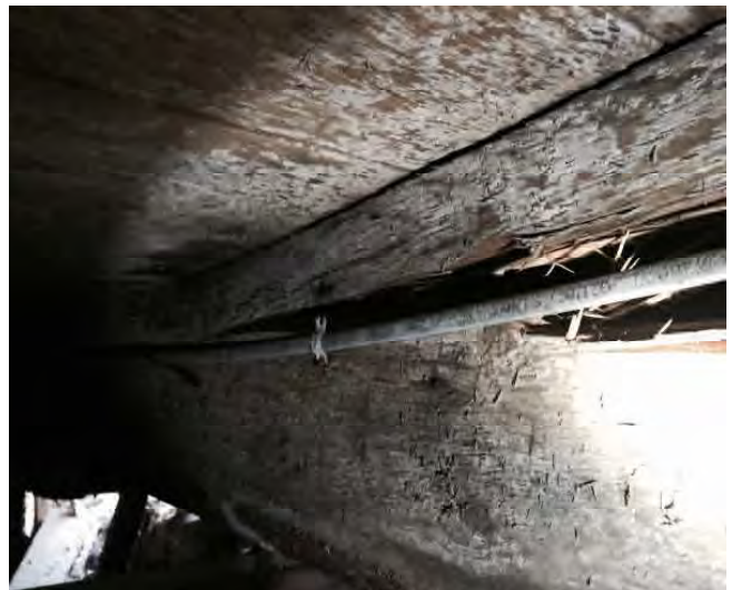
Cracked beam detail
