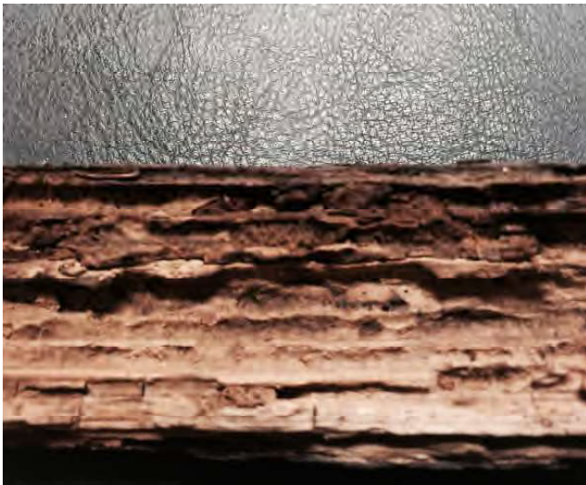
Wood worm attack of the beam
