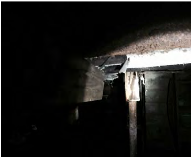
Beam supported by pipe
