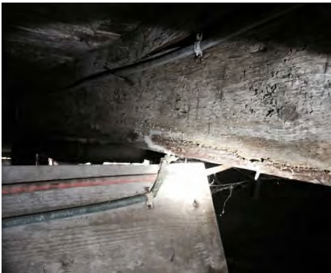
Cracked beam
