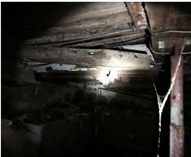
Beam supported by pipe
