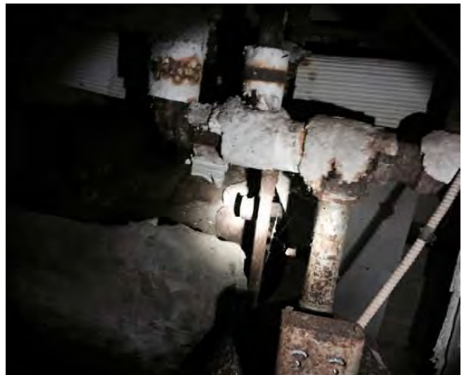
Furnace asbestos detail
