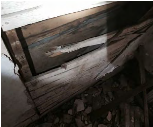
Main floor wall detail - mould
