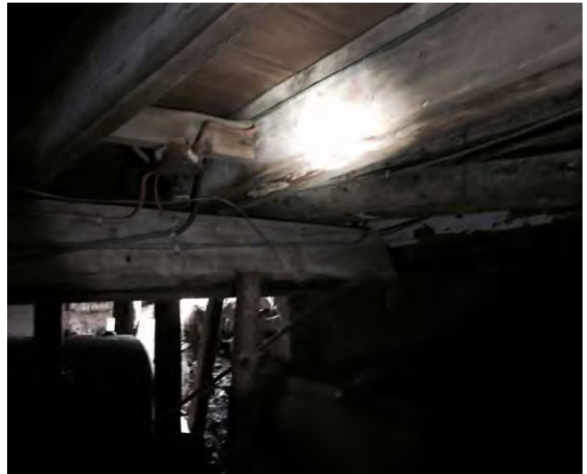
Beam lacking support
