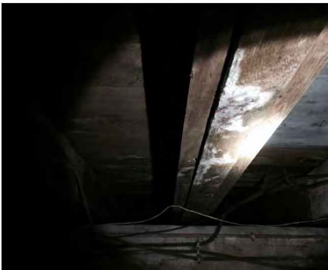
Beams with mould growth
