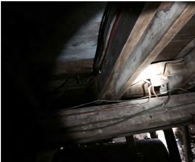
Beam lacking support
