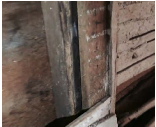
Main floor wall detail - mould
