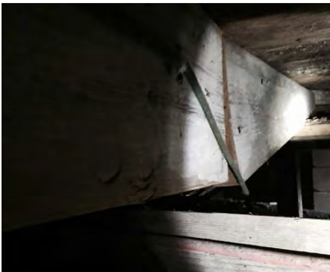
Cut beam, no support
