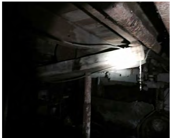
Loose beam supported by 1.5" pipe
