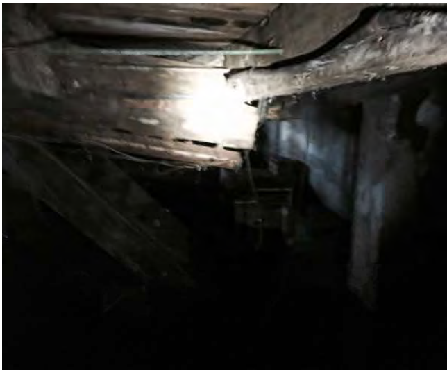
Unsupported beam detail
