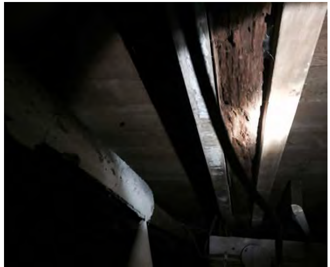
Original beam supported by 2" beams on each side
