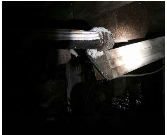
Asbestos detail
