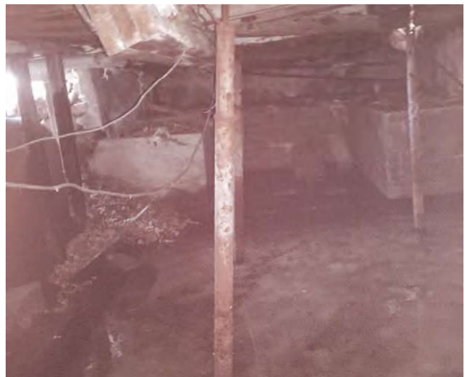
Basement pipe supports
