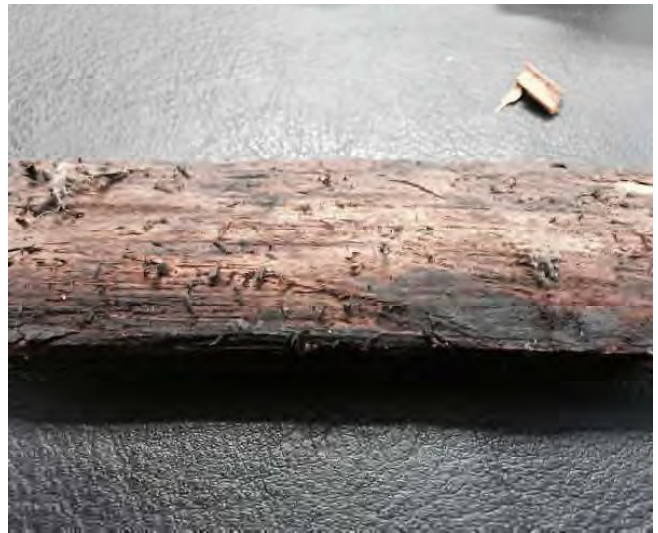
Mould and wood worm attack of the beam
