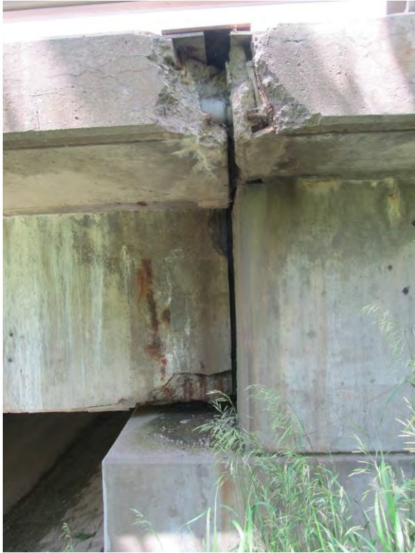
Exhibit 33 – Kennedy Rd – Rouge River Bridge Loss of Concrete under Northeast Expansion Joint (view from East)
