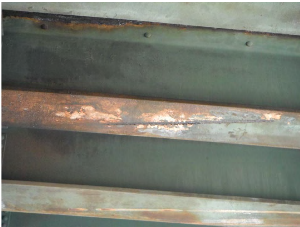
Corrosion on Girder
