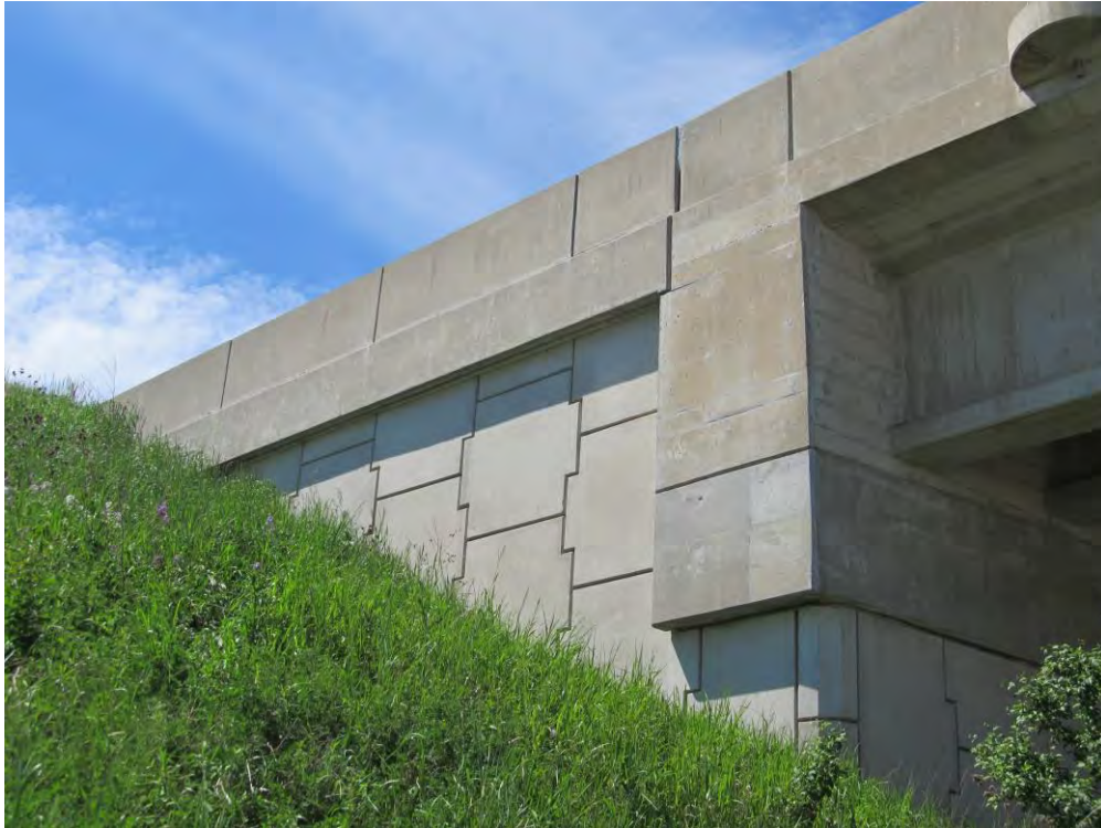
Exhibit 17 – Kennedy Rd – 407ETR Overpass Southeast Wingwall (view from Northeast)
