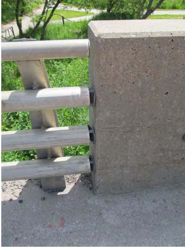
Exhibit 39 – Kennedy Rd – Rouge River Bridge Spalling & Loose End Caps on Southeast Railing (view from West)
