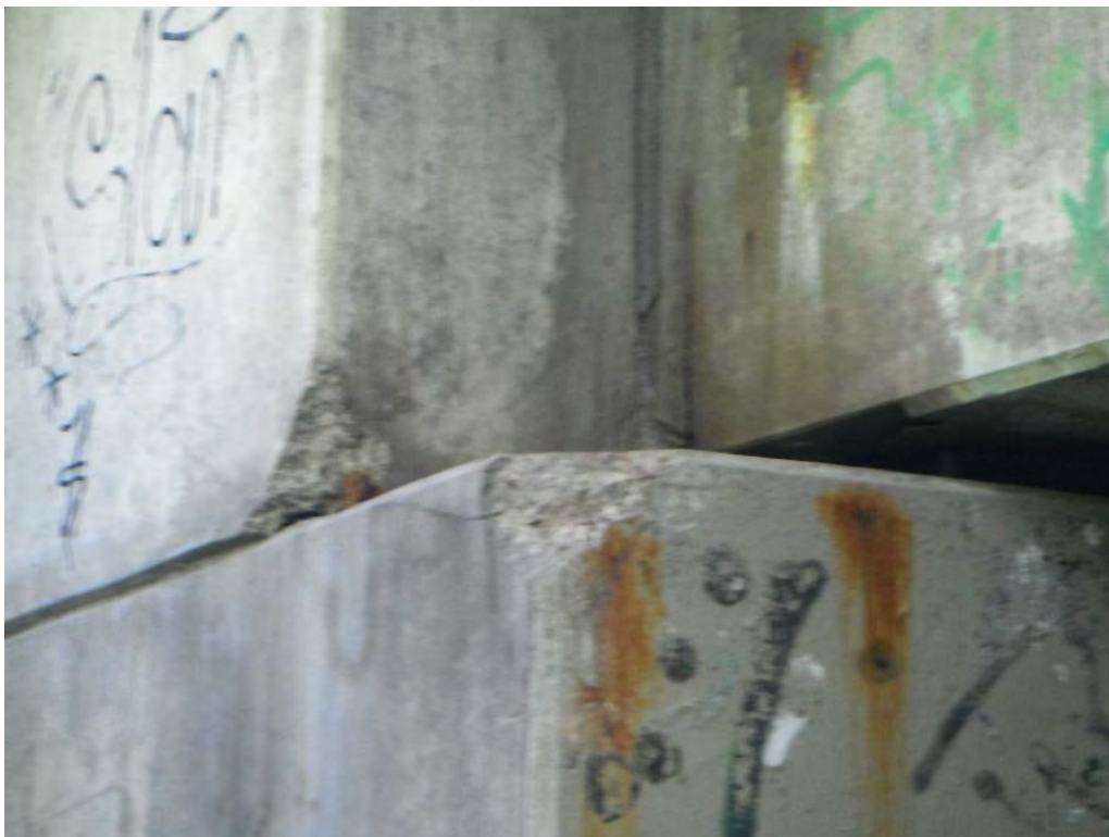
Spall on Abutment and Ballast Wall
