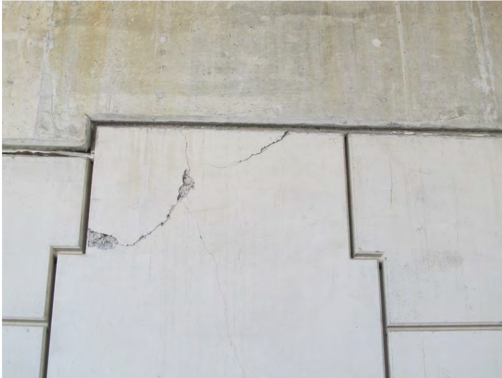
Exhibit 15 – Kennedy Rd – 407ETR Overpass Delamination on Southeast Abutment (view from North)
