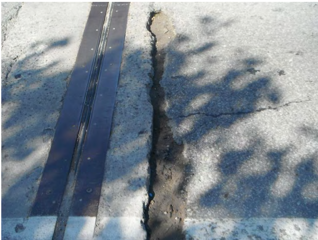
Pot Hole Adjacent to North Expansion Joint
