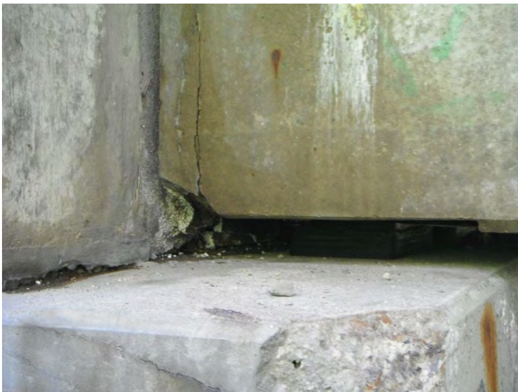
Spall on Girder End
