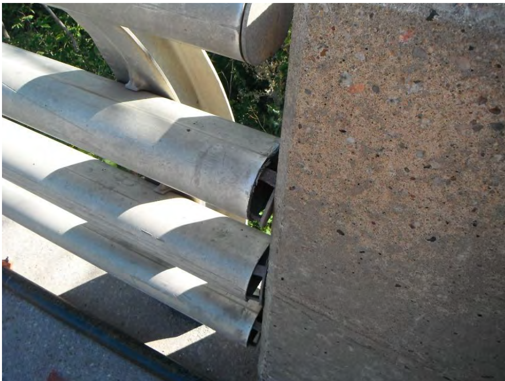
Bent and Broken End Caps
