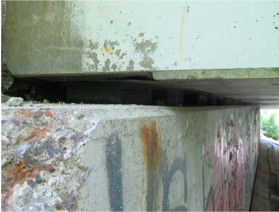
Exhibit 31 – Kennedy Rd – Rouge River Bridge Spalling on Northwest Bearing Seat (view from West)
