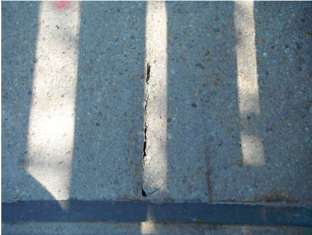
Medium Crack on Concrete End Dam
