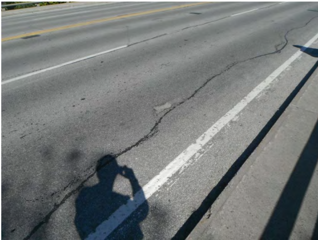
Sealed Crack on Deck Surface
