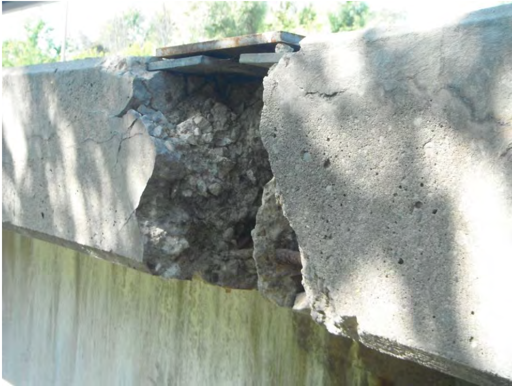
Spall and Exposed Rebar at Expansion Joint
