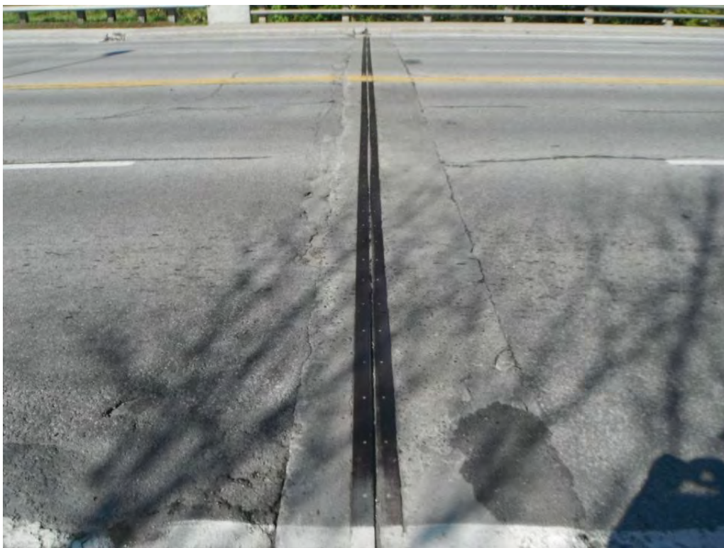
Pot Holes at South Expansion Joint
