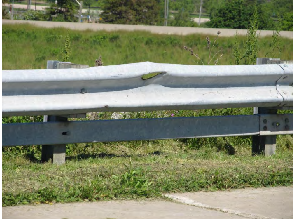
Exhibit 26 – Kennedy Rd – 407ETR Overpass Damage on Southwest Guiderail (view from East)
