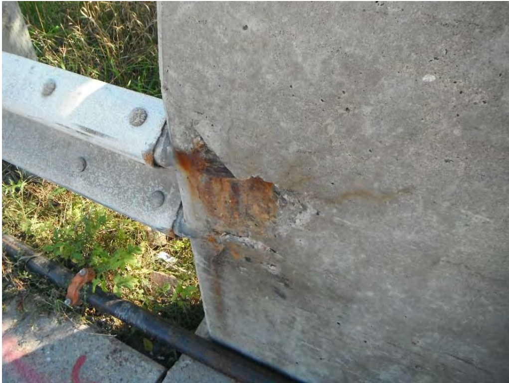
Spall on Interior Barrier Wall
