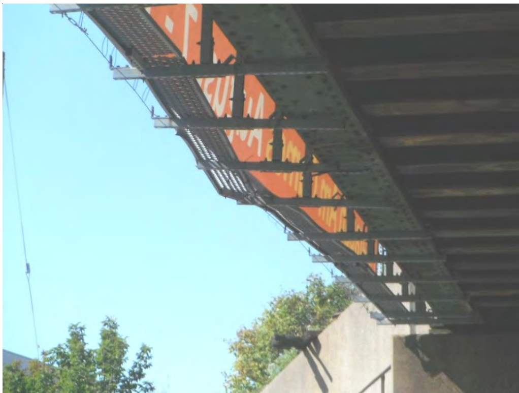
Vehicle Strike Damage on Sign
