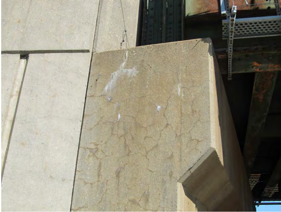
Exhibit 07 – Kennedy Rd – CN Rail Underpass Map Cracks and Efflorescence on Southwest Bearing Seat (view from South)
