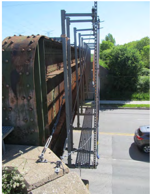
Exhibit 08 – Kennedy Rd – CN Rail Underpass South Exterior Girder & Trainmen's Walk, Missing Sections (view from West)
