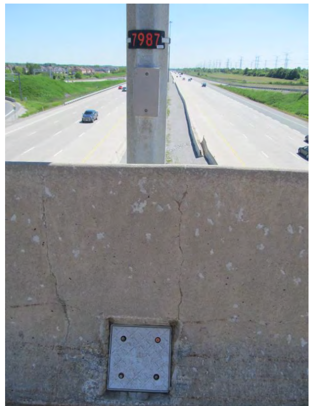
Exhibit 24 – Kennedy Rd – 407ETR Overpass Cracks & Spalls on East Barrier Wall at Middle Light Pole (view from West)
