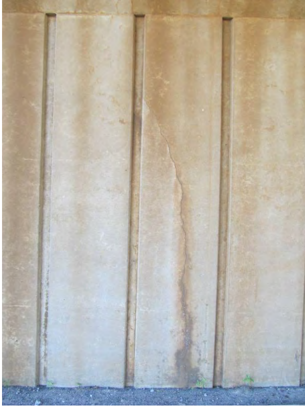
Exhibit 03 – Kennedy Rd – CN Rail Underpass Wide Crack on East Abutment, Base of Middle Portion (view from West)
