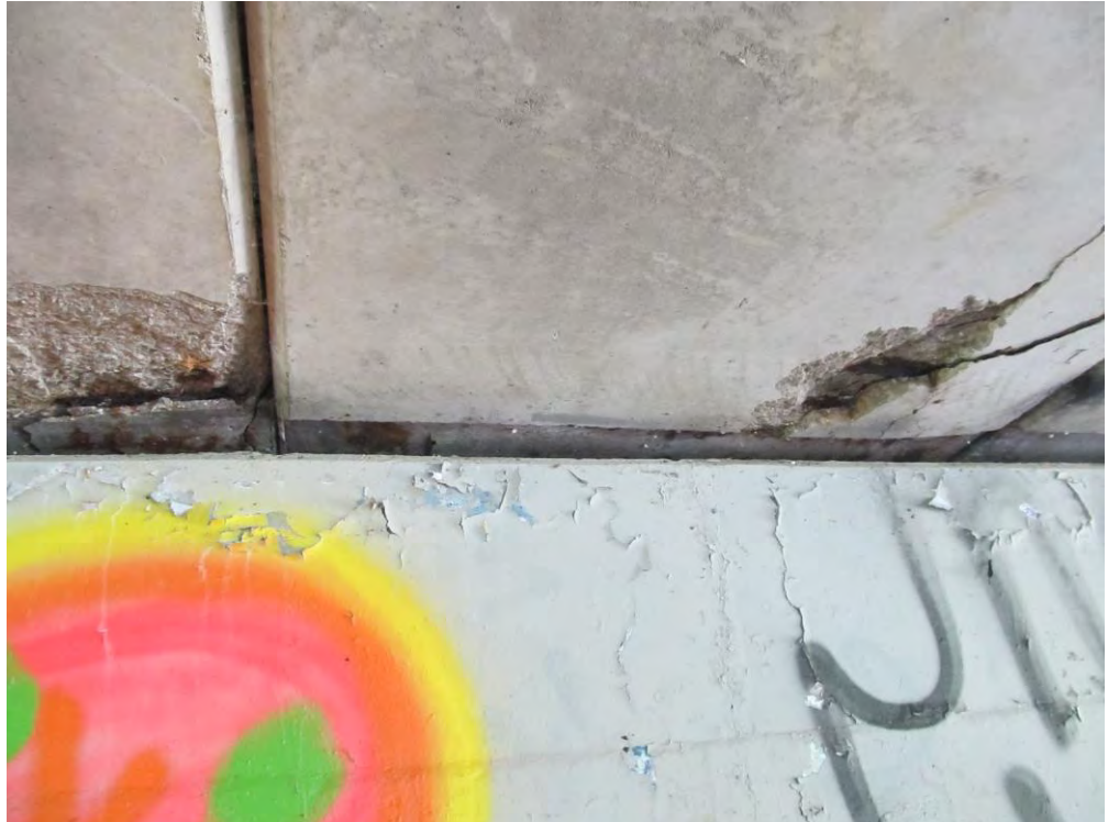
Exhibit 30 – Kennedy Rd – Rouge River Bridge Delamination & Exposed Rebar on North End of Soffit (view from South)
