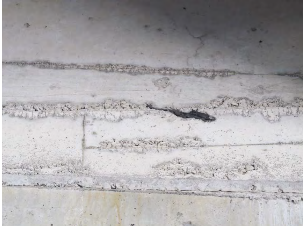
Exhibit 16 – Kennedy Rd – 407ETR Overpass Concrete Segregation on North Abutment, Top of Middle Portion (view from South)
