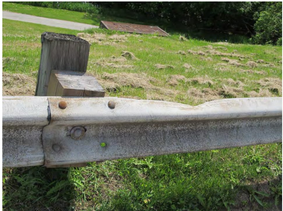
Exhibit 40 – Kennedy Rd – Rouge River Bridge Dent & Missing Bolt on Northeast Guiderail (view from West)
