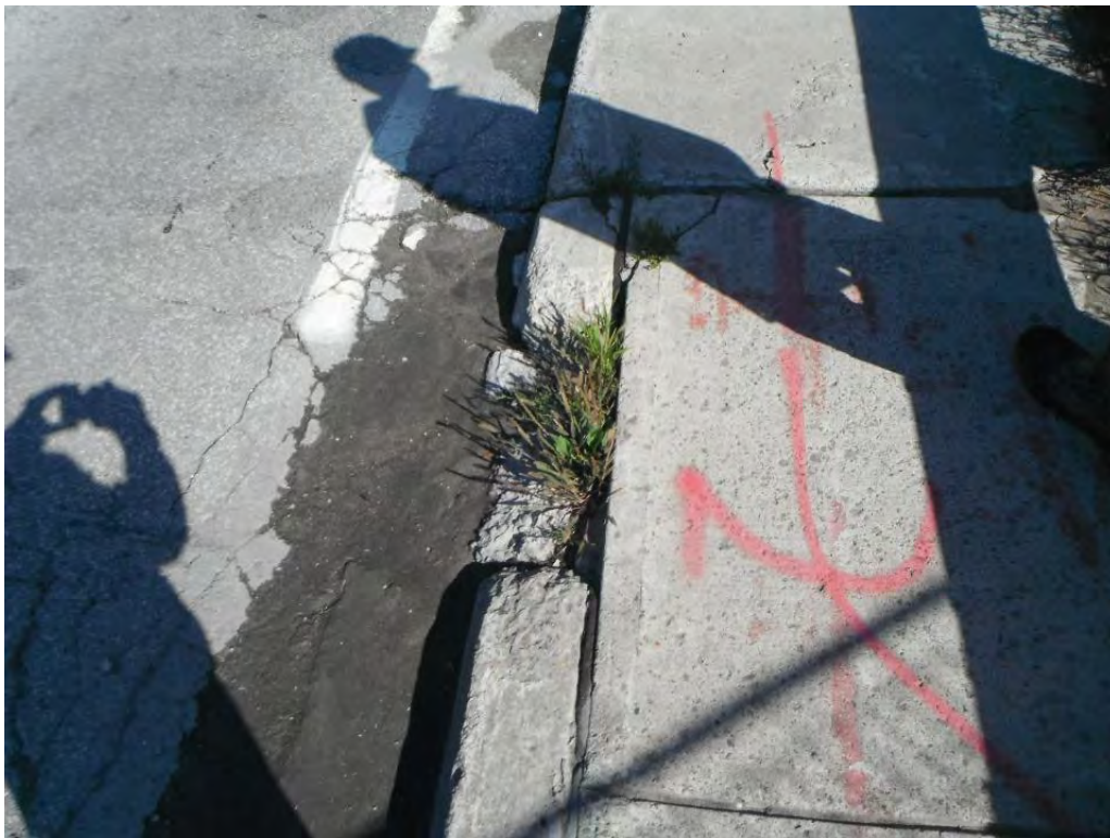
Severe Spall on Curb
