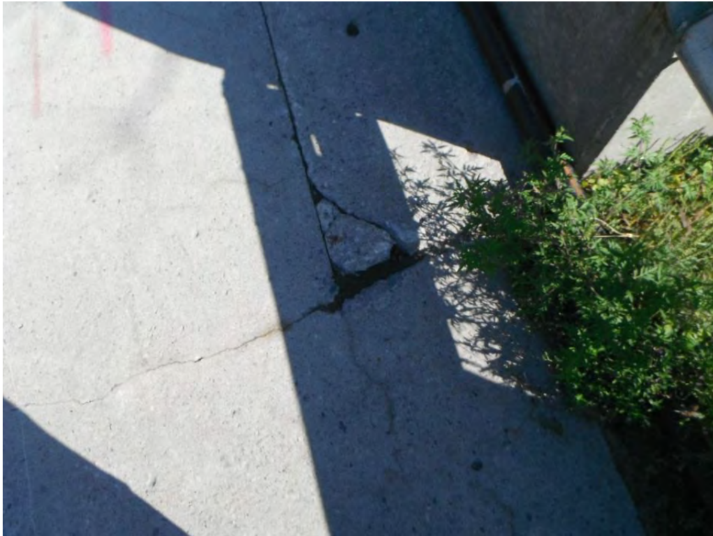
Spall on Sidewalk
