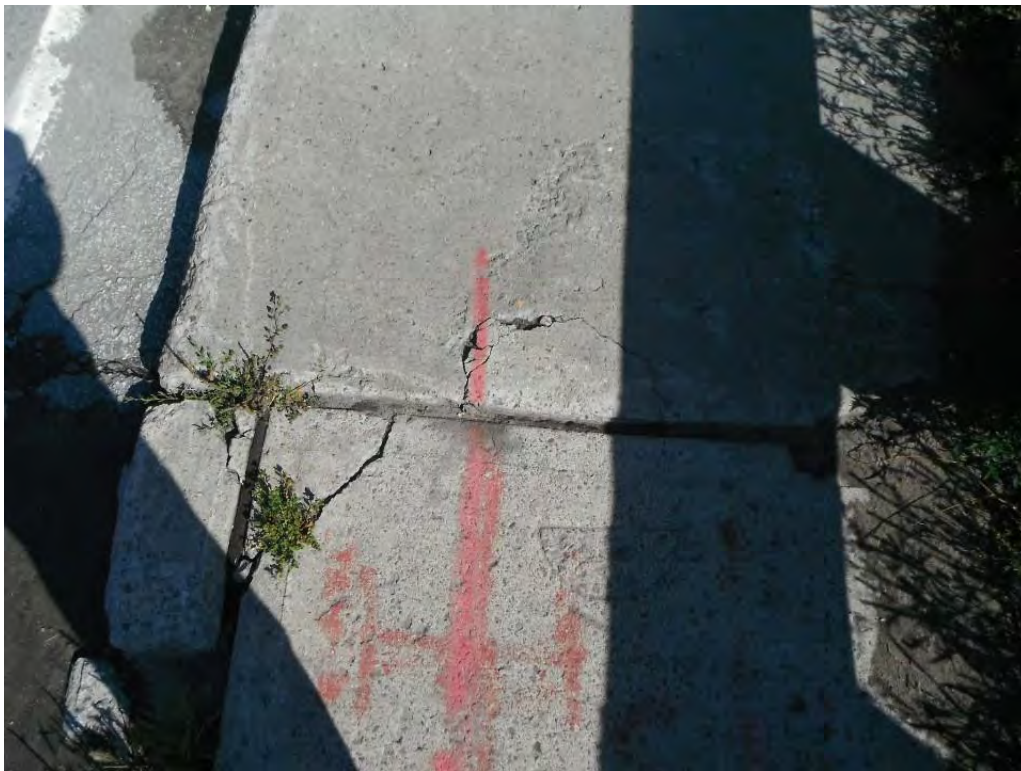
Medium Cracks on Sidewalk
