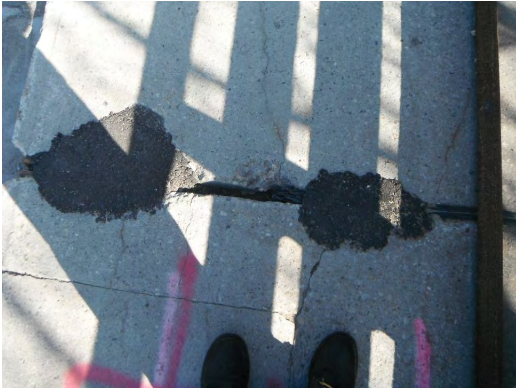
Spall on Sidewalk
