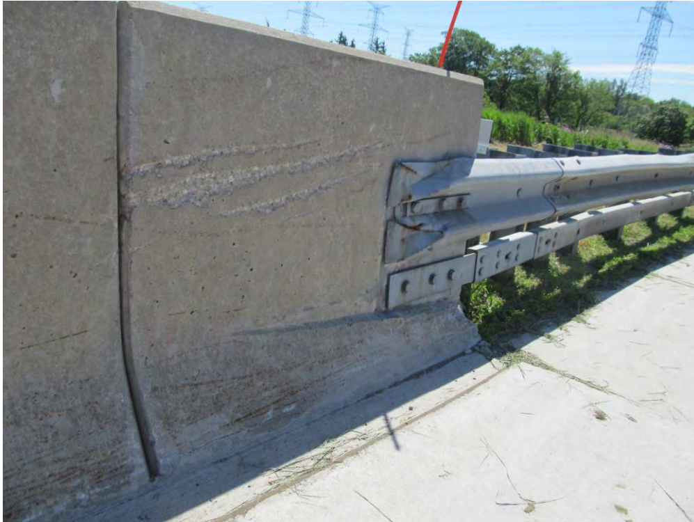
Exhibit 25 – Kennedy Rd – 407ETR Overpass Impact Damage at Southeast Barrier Wall/Guiderail Connection (view from North)
