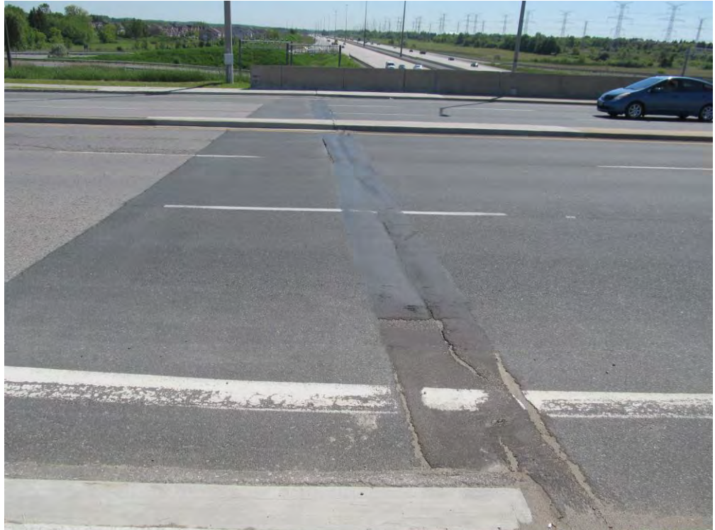
Exhibit 20 – Kennedy Rd – 407ETR Overpass Cracks and Deterioration on North Approach (view from West)
