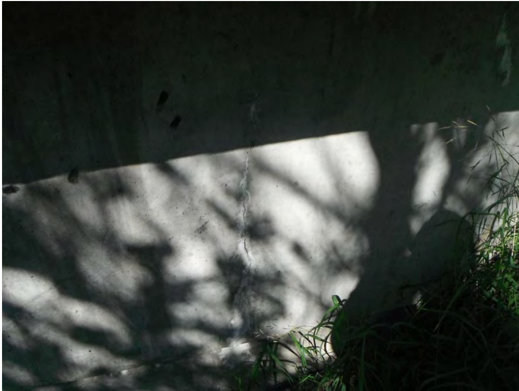
Crack on Northeast Wingwall
