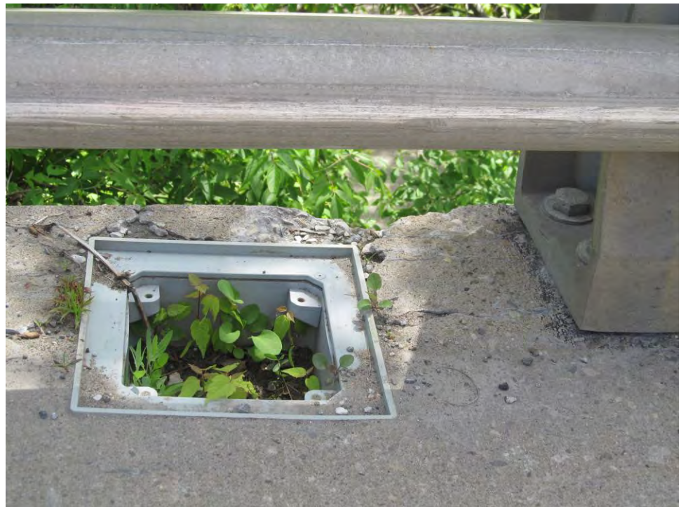
Exhibit 38 – Kennedy Rd – Rouge River Bridge Spall & Missing Cover from Northeast Electrical Box (view from West)
