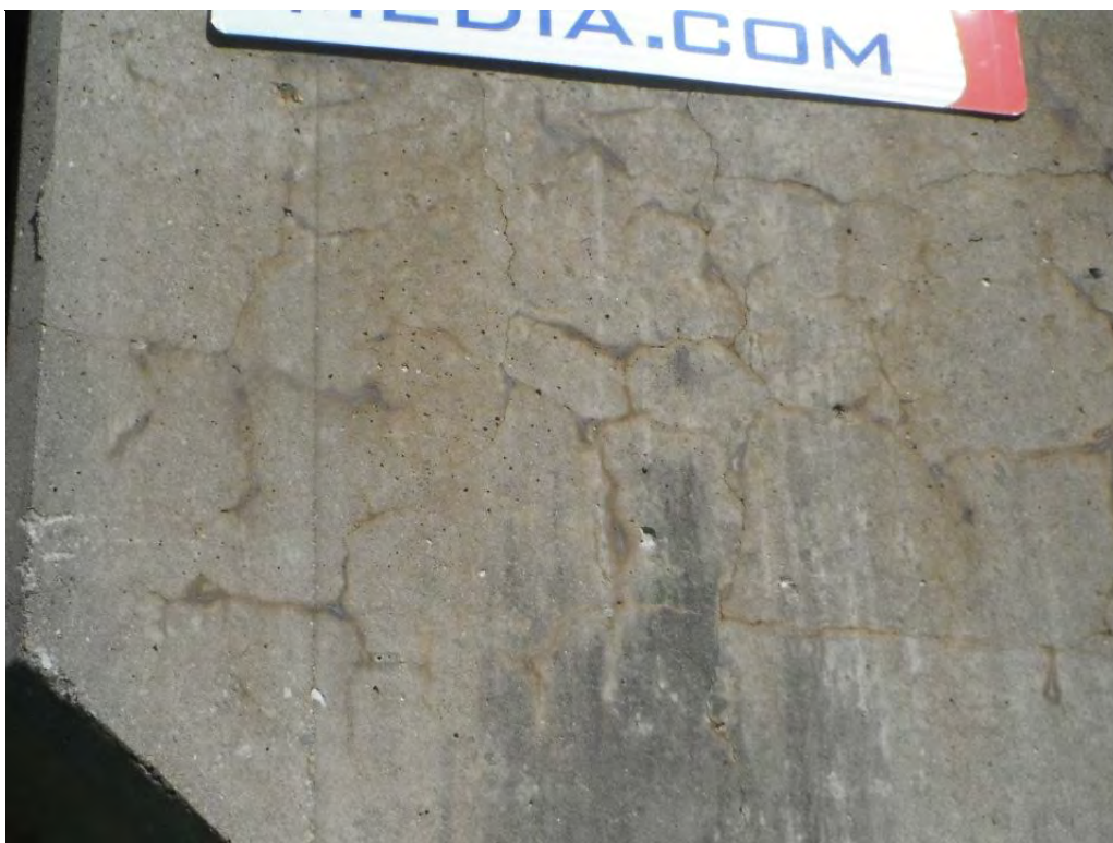
Map Cracking on Wingwall
