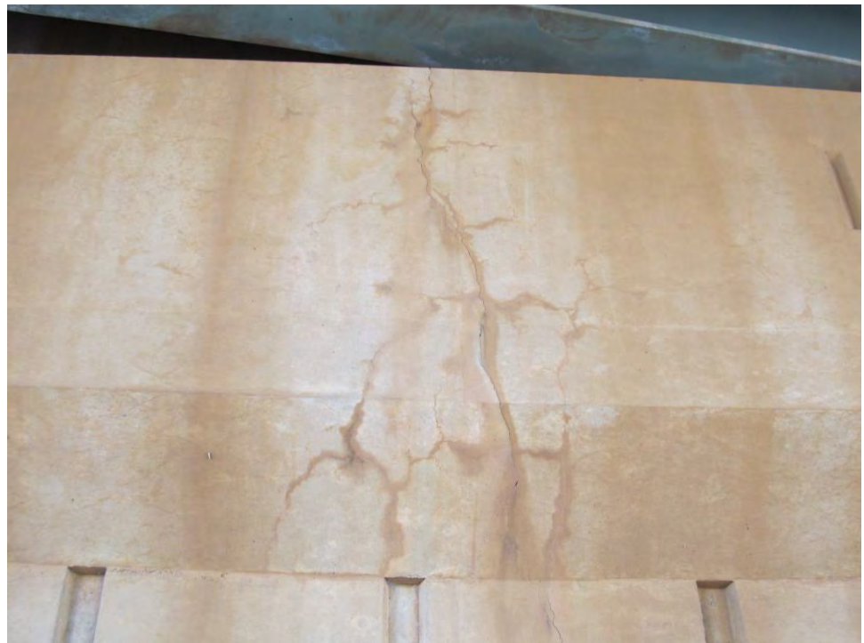
Exhibit 04 – Kennedy Rd – CN Rail Underpass Wide & Map Cracking on East Abutment, Top of Middle Portion (view from West)
