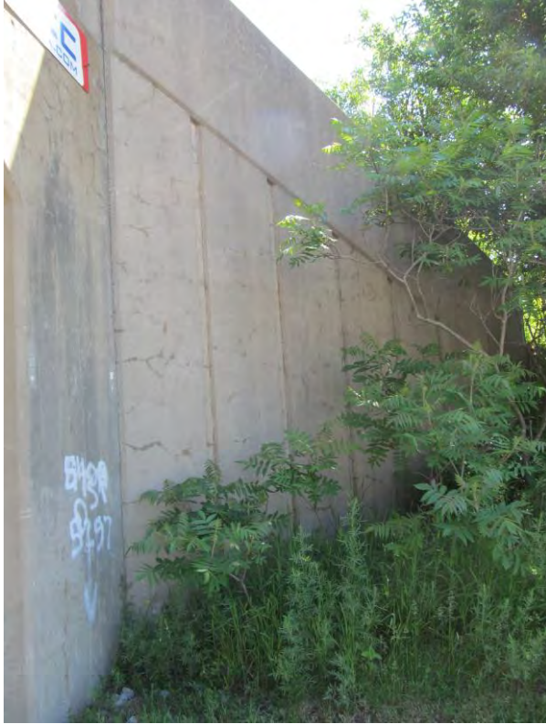
Exhibit 05 – Kennedy Rd – CN Rail Underpass Stained Map Cracks on Southeast Wingwall (view from Southwest)
