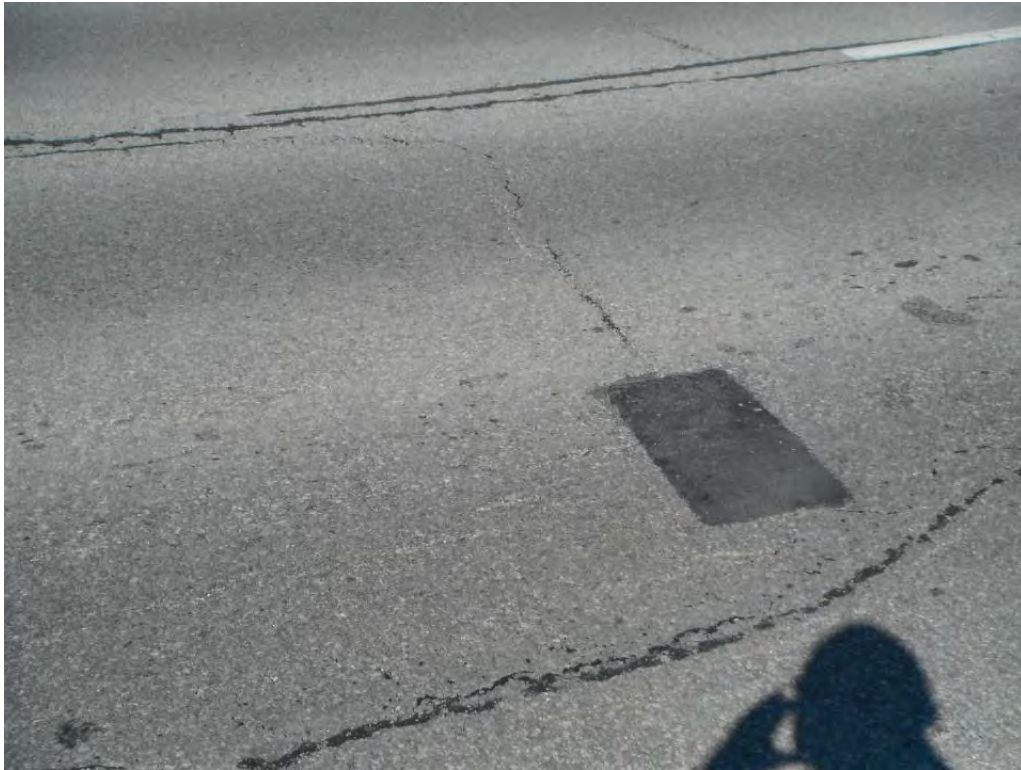
Sealed and Unsealed Cracks on Surface
