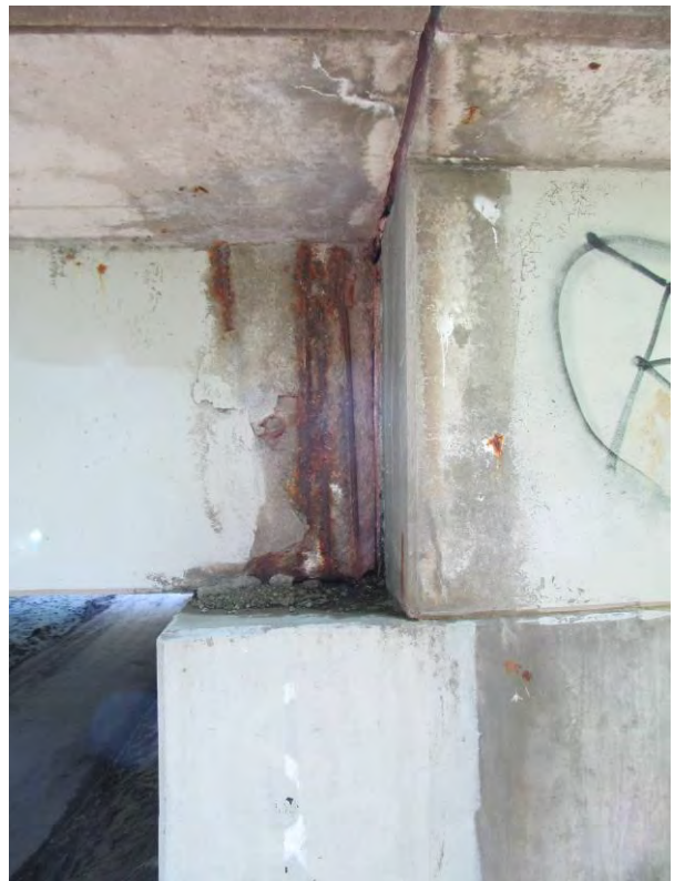
Exhibit 32 – Kennedy Rd – Rouge River Bridge Exposed Rebar on Southwest Girder End (view from West)
