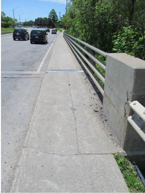
Exhibit 37 – Kennedy Rd – Rouge River Bridge West Sidewalk & Railing, Cracks & Spalling (view from North)
