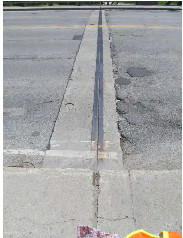
Exhibit 36 – Kennedy Rd – Rouge River Bridge South Expansion Joint, Cracks/Deterioration/Patches (view from West)
