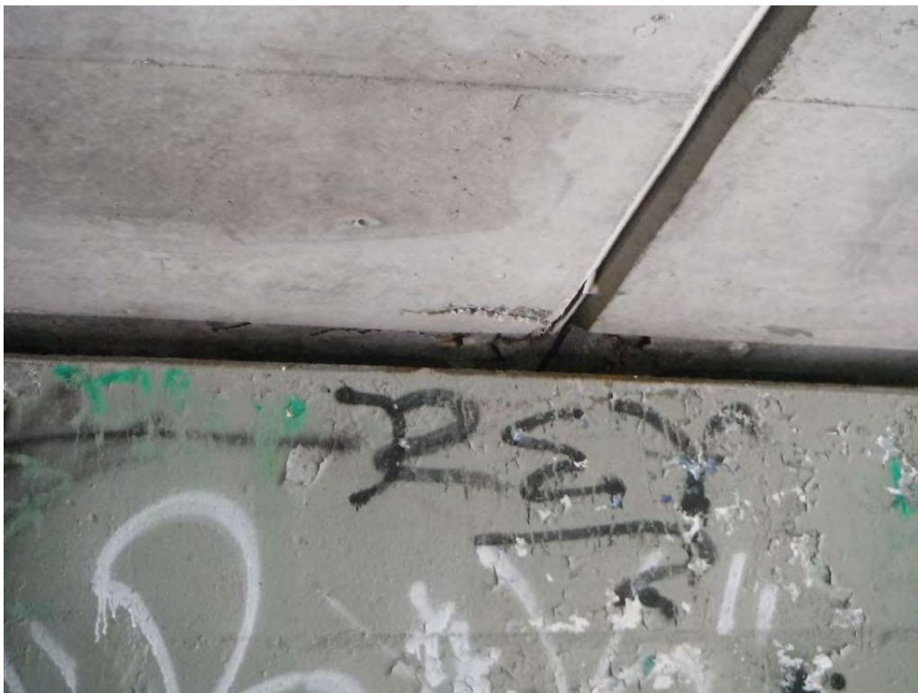
Delamination on Girder End
