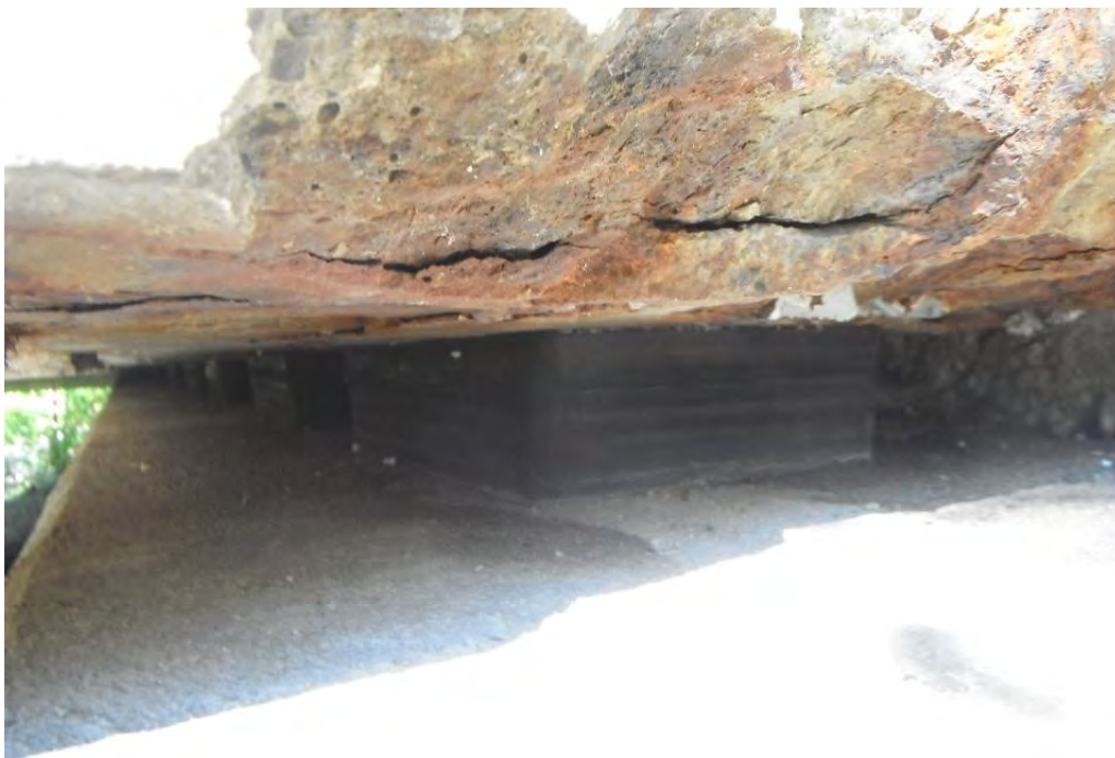
Spall on Abutment and Ballast Wall
