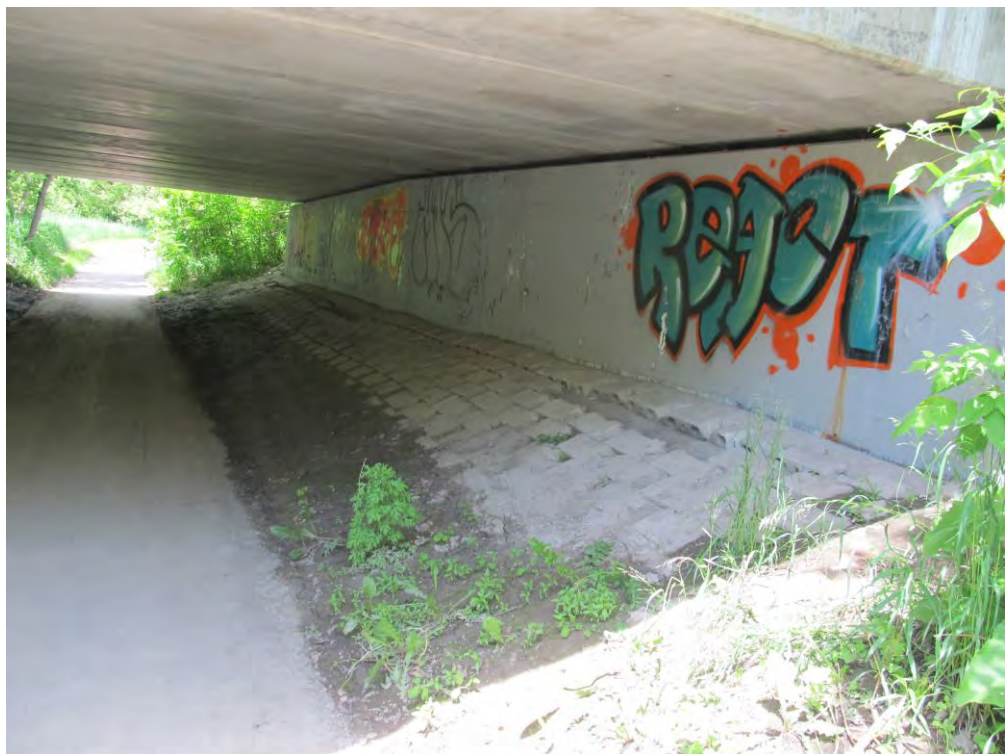
Exhibit 28 – Kennedy Rd – Rouge River Bridge North Abutment, Graffiti & Missing Slope Protection Blocks (view from Southeast)
