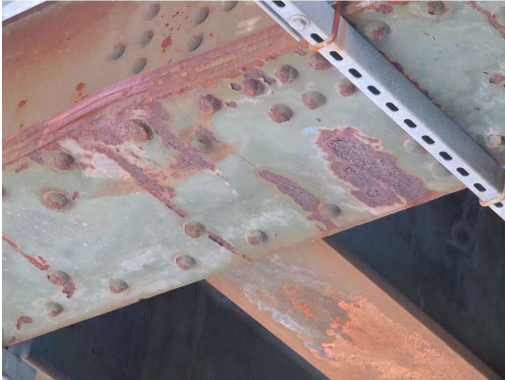
Exhibit 11 – Kennedy Rd – CN Rail Underpass Impact Damage on Bottom Flange of Southeast Girder (view from Southeast)
