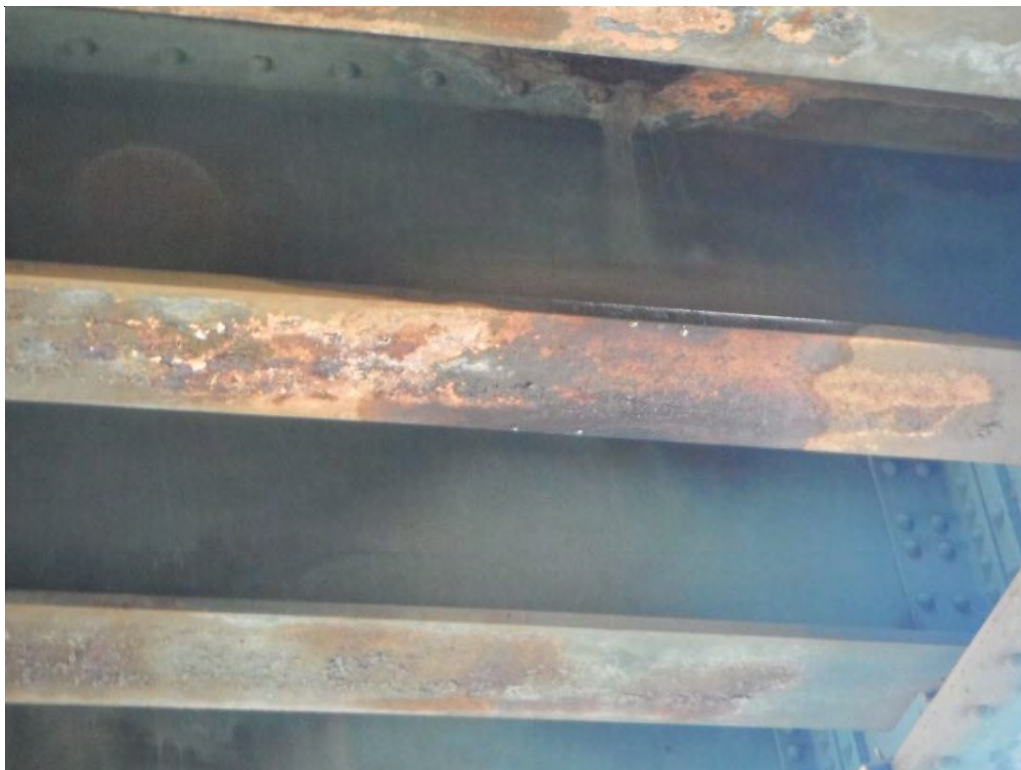
Corrosion on Girder
