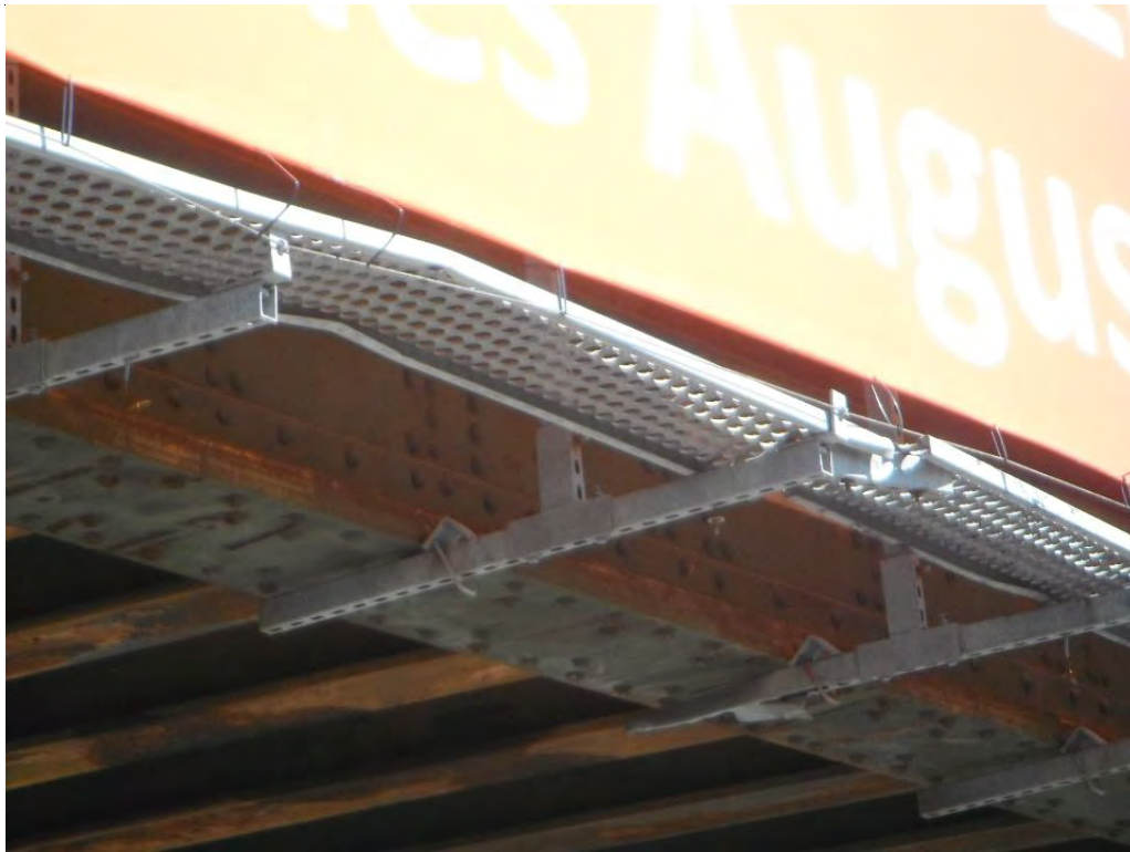
Vehicle Strike Damage on Exterior Sign
