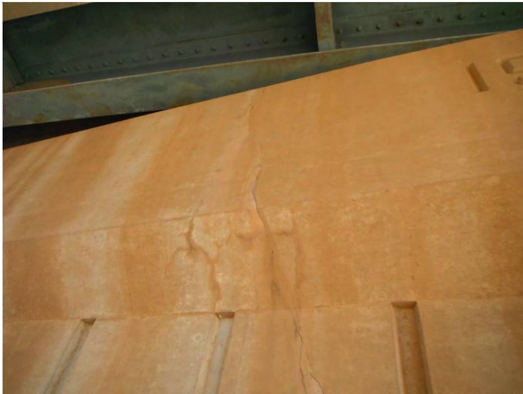
Crack on Abutment
