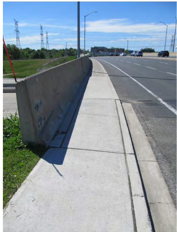
Exhibit 22 – Kennedy Rd – 407ETR Overpass Missing Guiderail at Southeast Barrier Wall & Sidewalk (view from North)
