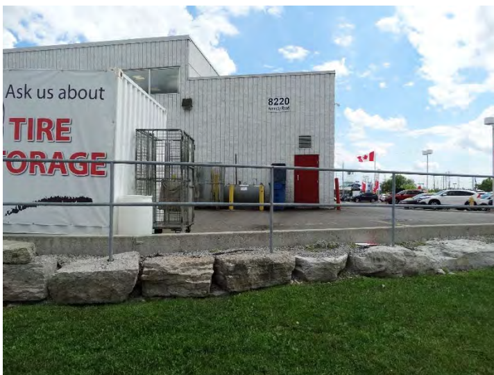
Photo 8 - View of ethylene glycol tank at Markham Honda at 8220 Kennedy Road (Section 2, facing south).
