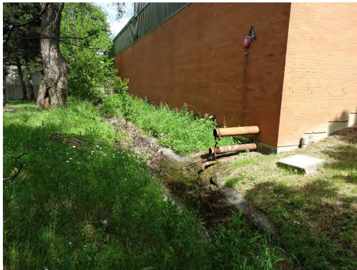
Photo 4 - View of three of the four outfalls to drainage channel at Bell, 7733 Kennedy Road (Section 1, facing east).
