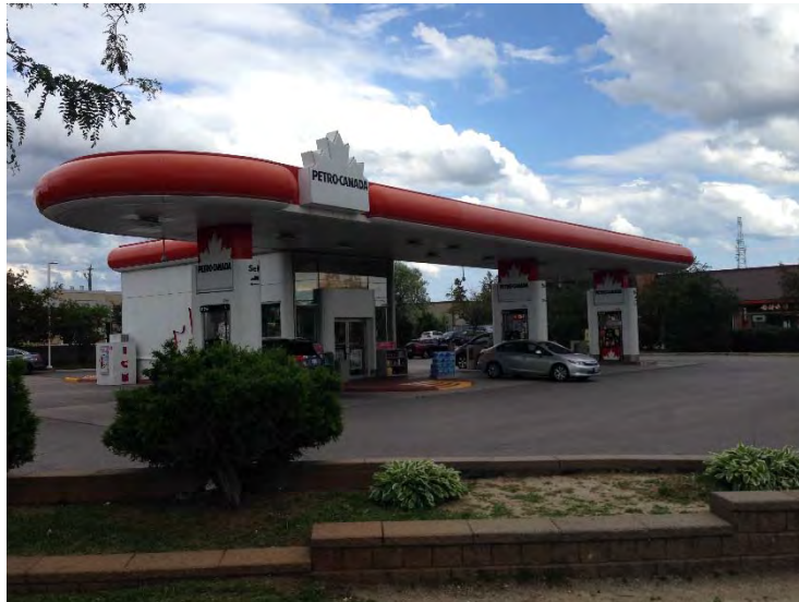
Photo 2 - View of Petro Canada retail service station at 4575 Steeles Ave East (Section 1, facing east).
