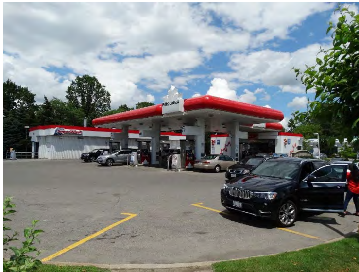
Photo 14 - View of Petro Canada Gas Station at 4780 Highway 7 (Section 3, facing northwest).
