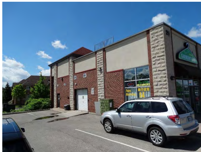
Photo 2 – Garment Care dry cleaners at 20 Bur Oak Ave (Section 4, facing south-west).
