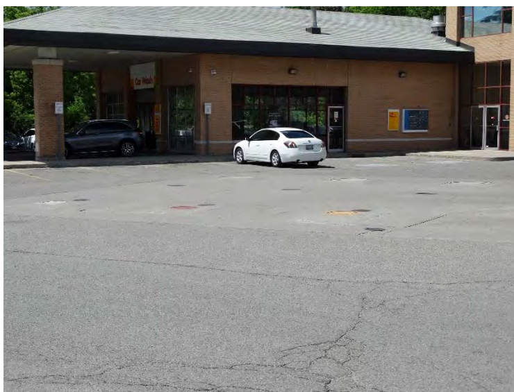
Photo 7 – View of tank lids at Shell Retail Gas Station at 8338 Kennedy Road (Section 2, facing west)
