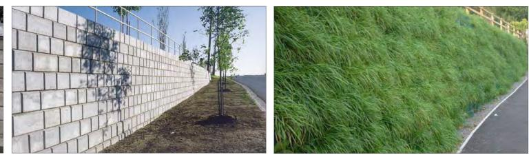
Pedestrian Retaining Wall Option: 200mm-1200mm Engineered Retaining Wall Option: 1200mm +
