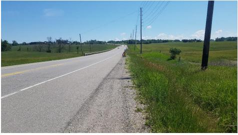
Image 9: Forcemain – View of disturbances associated with previous roadway improvements (drainage ditching, traffic barrier, asphalt and gravel shoulders, built-up grassed margins).
