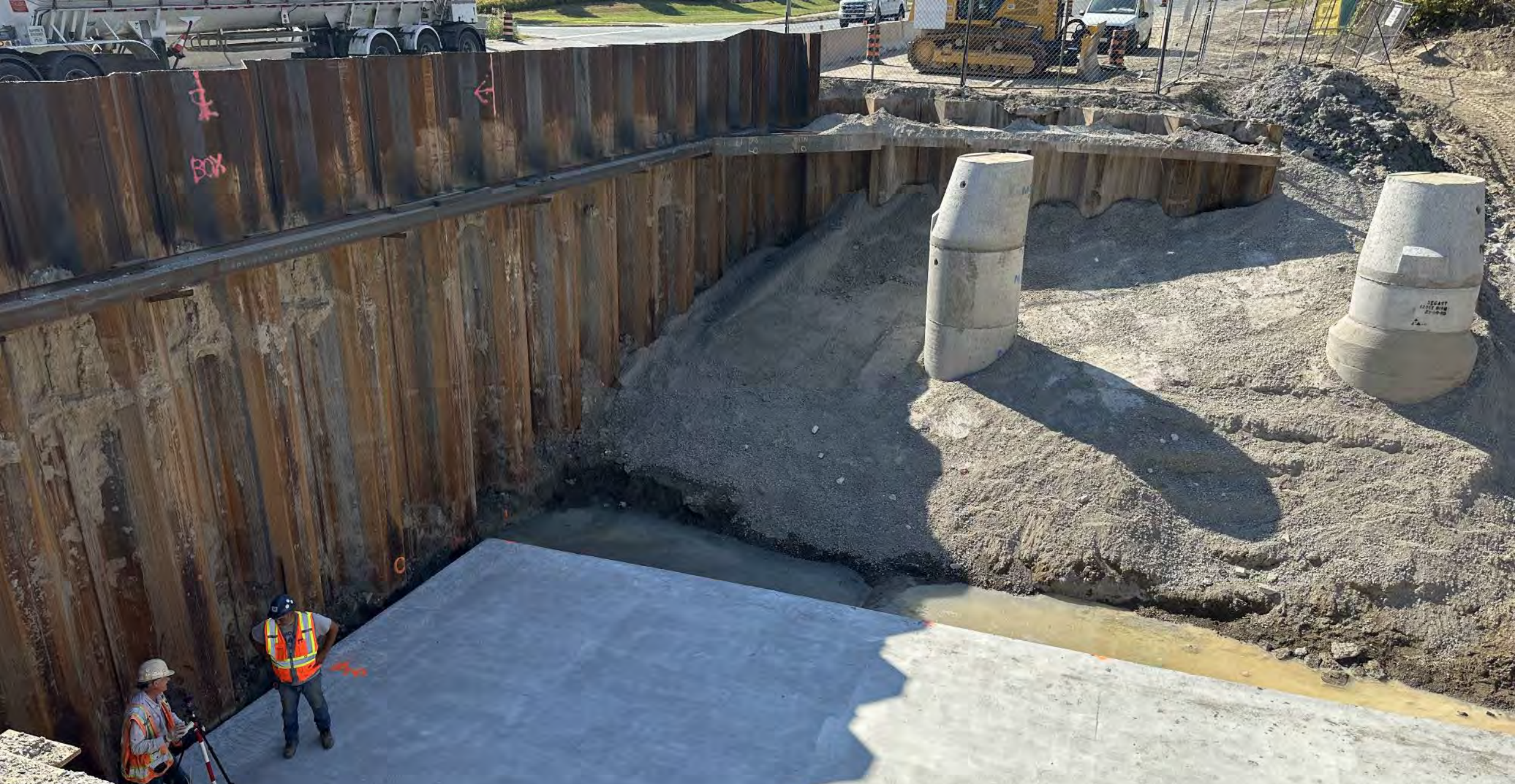
Concrete slab to support culvert
