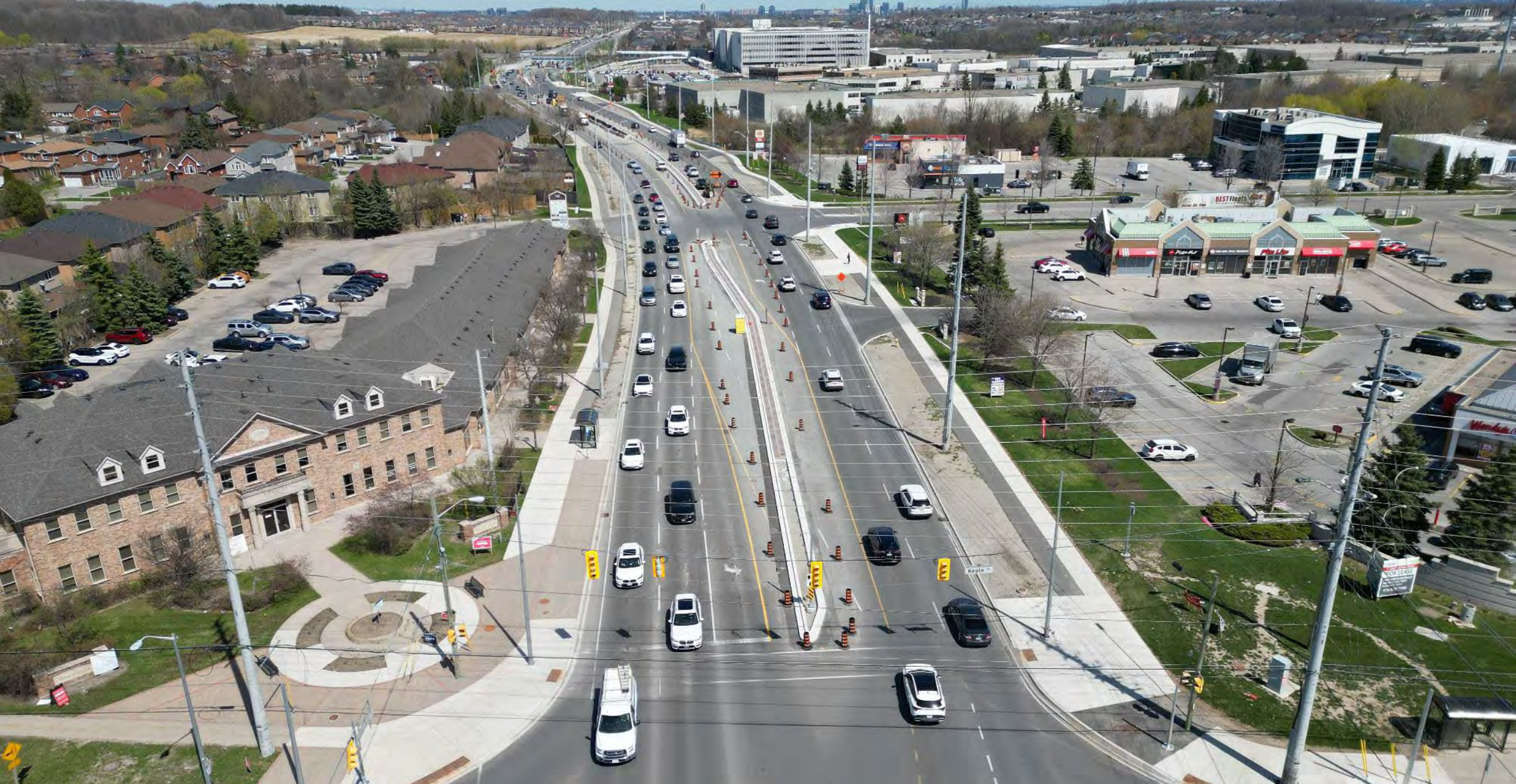
Widened road and new median, Rutherford Road, east of Keele Street
