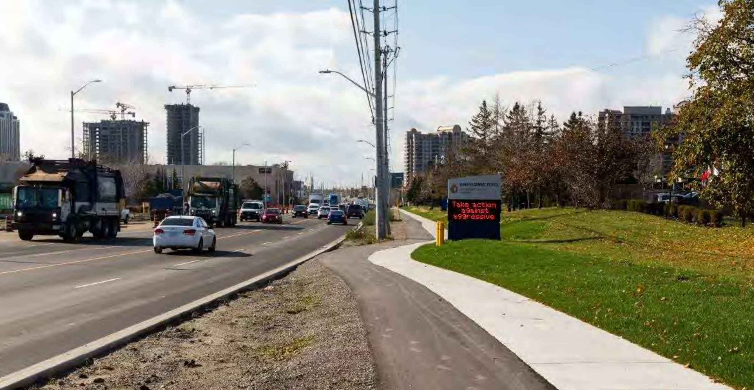
New sidewalks and cycle tracks on Rutherford Road
