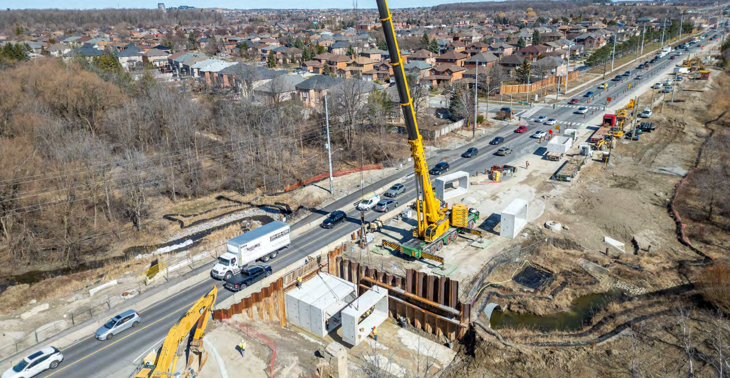
Installation of new culvert on Rutherford Road, west of Greenock Drive
