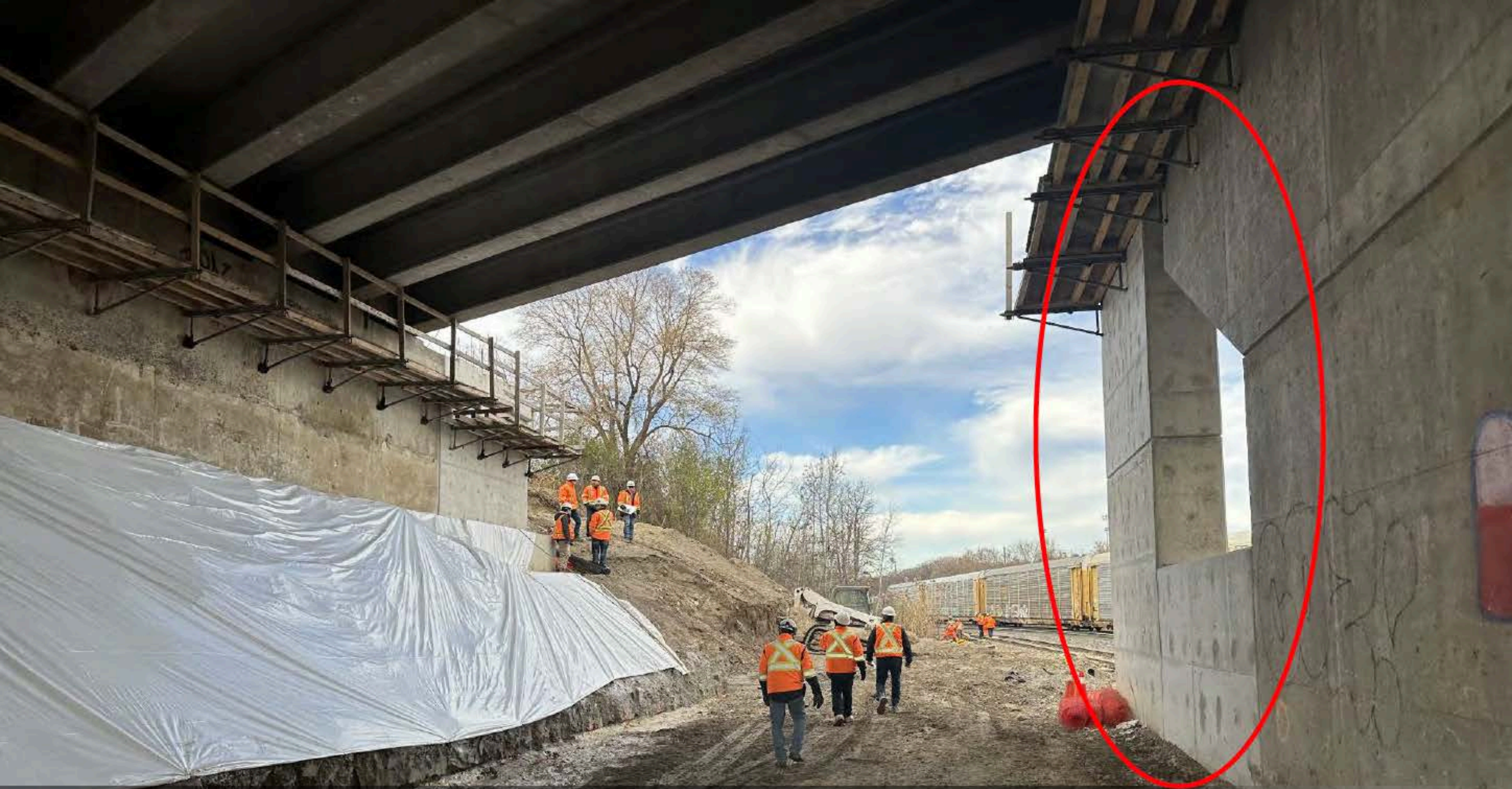
New west pier of Rutherford Road bridge over CN Rail tracks
