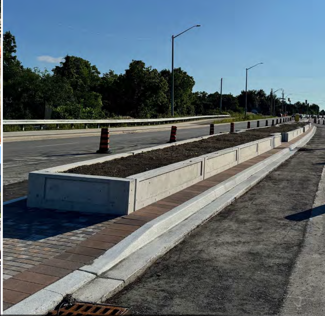
Medians are being installed to reduce the risk of serious collisions, increase pedestrian safety and provide streetscaping
