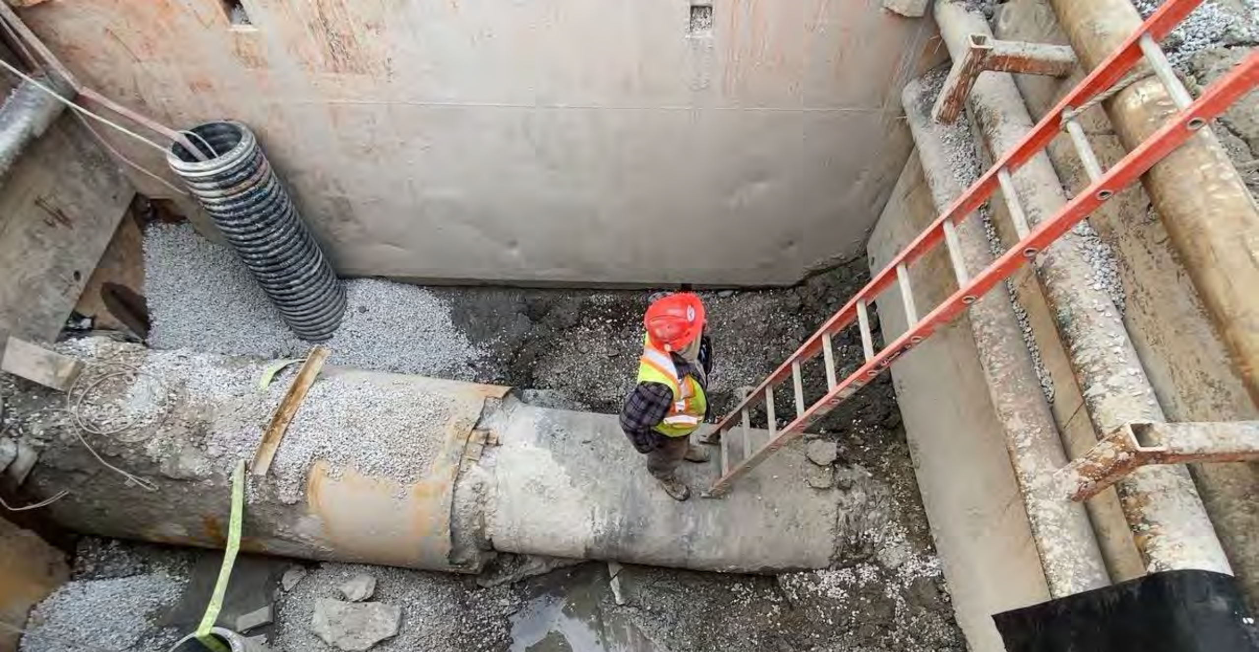
Construction of watermain protection under CN Rail bridge on Rutherford Road
