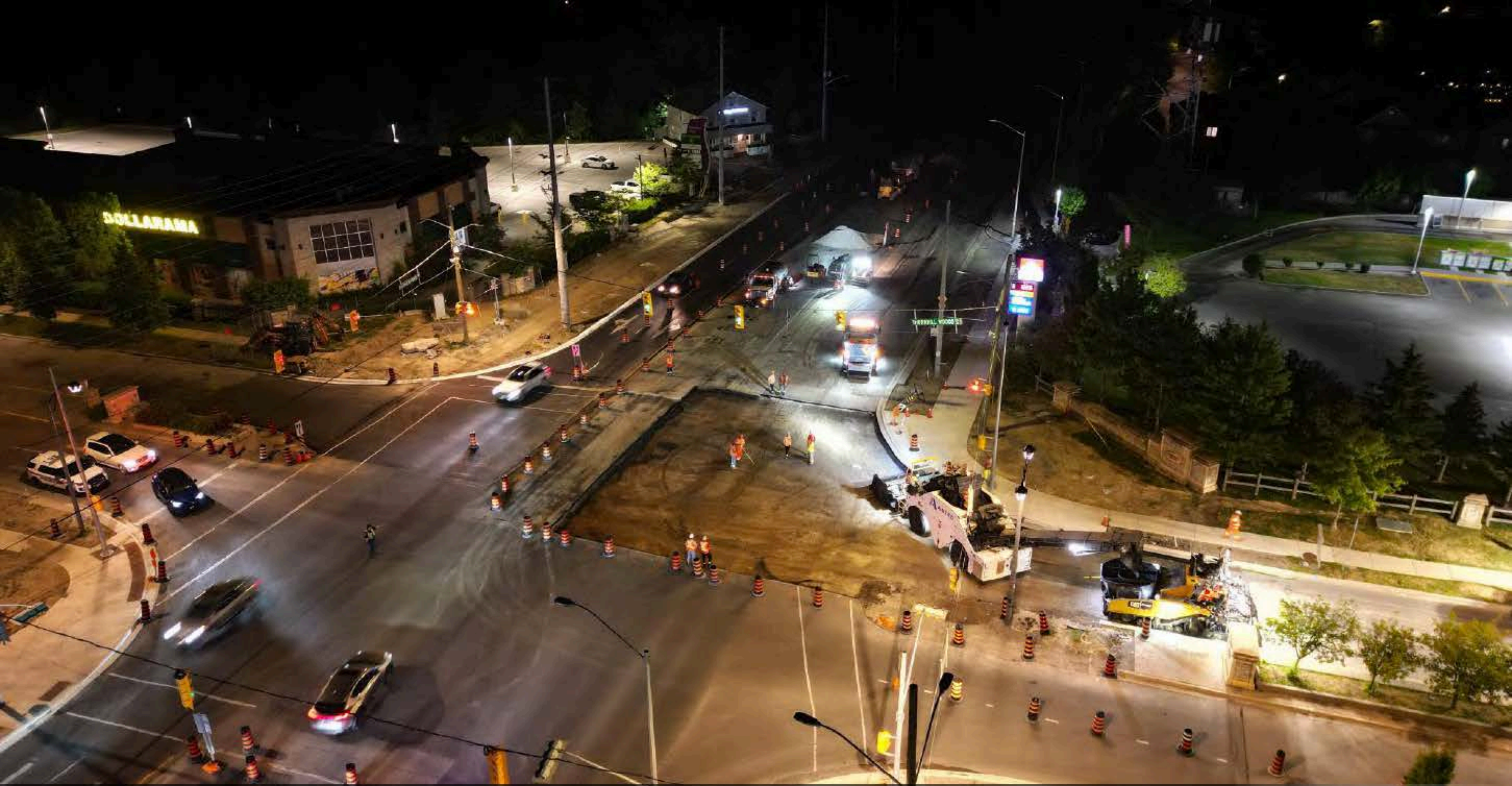
Night paving on Rutherford Road at Thornhill Woods Drive
