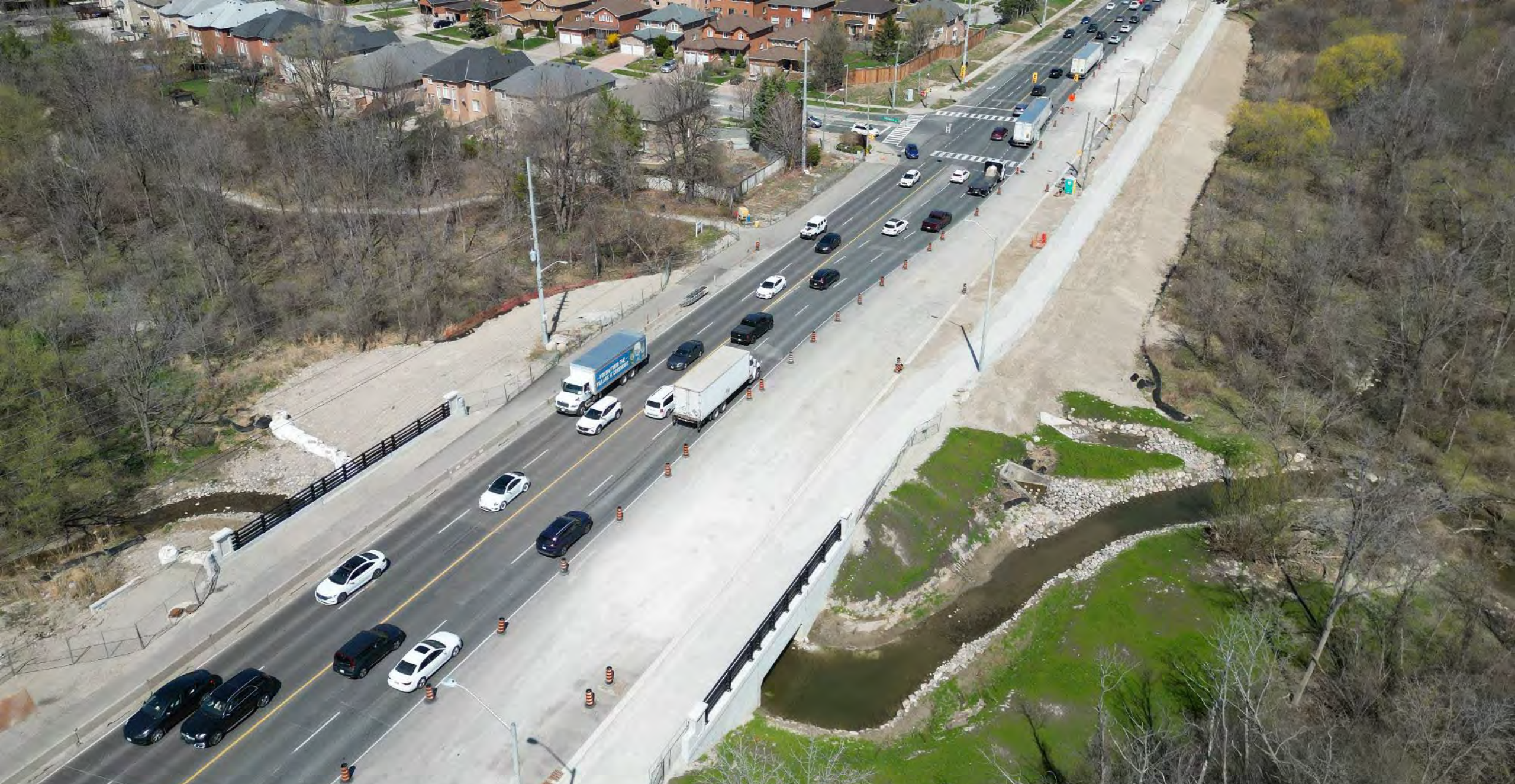
Completed culvert on Rutherford Road, west of Greenock Drive
