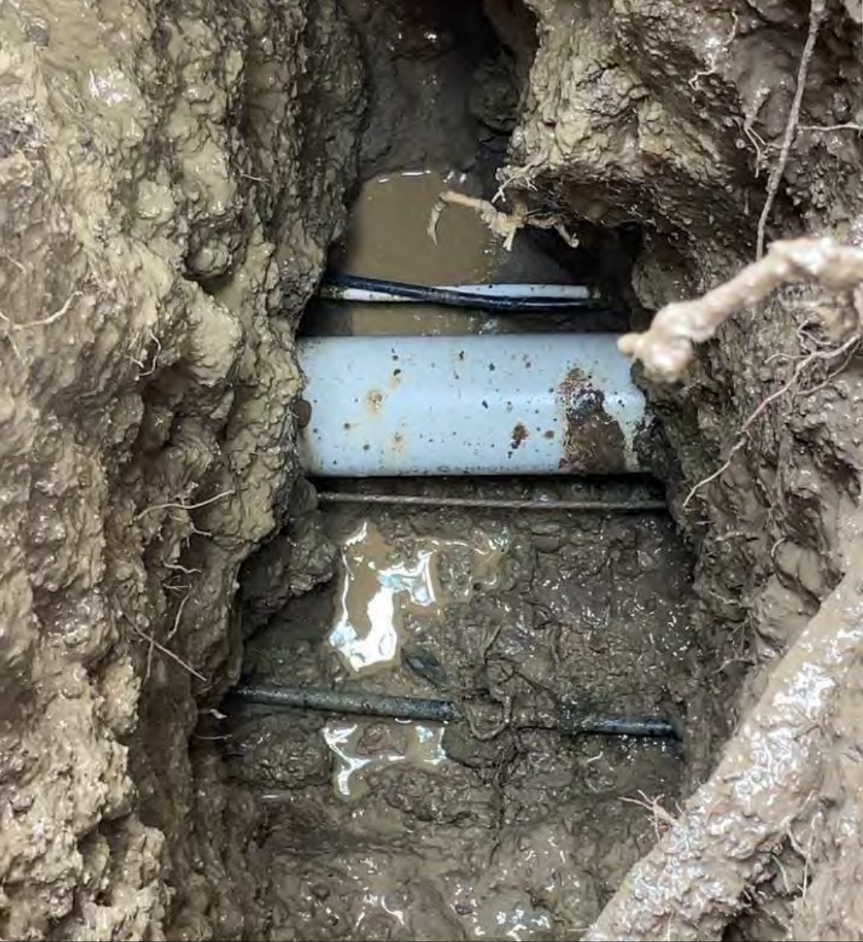
Unexpected utility conflicts discovered during construction
