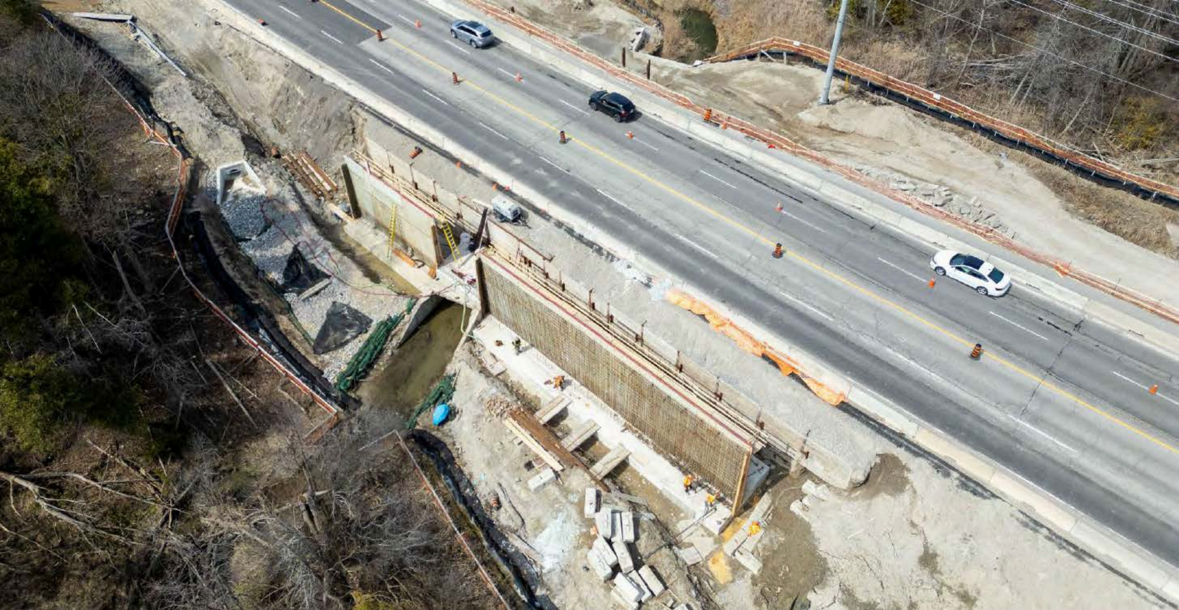
Preparation for installation of culvert extension on Rutherford Road
