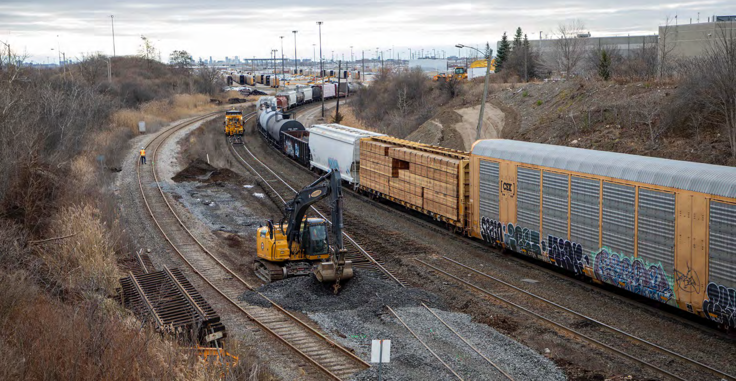
CN track realignment to allow for bridge widening on Rutherford Road
