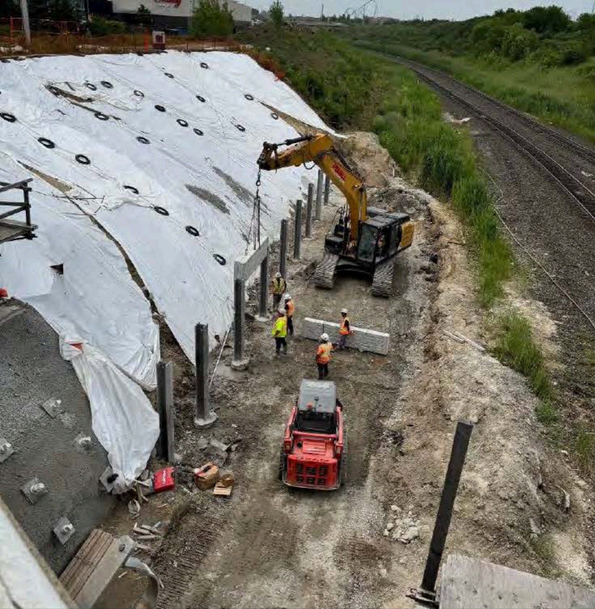
Retaining wall construction under CN Rail bridge on Rutherford Road
