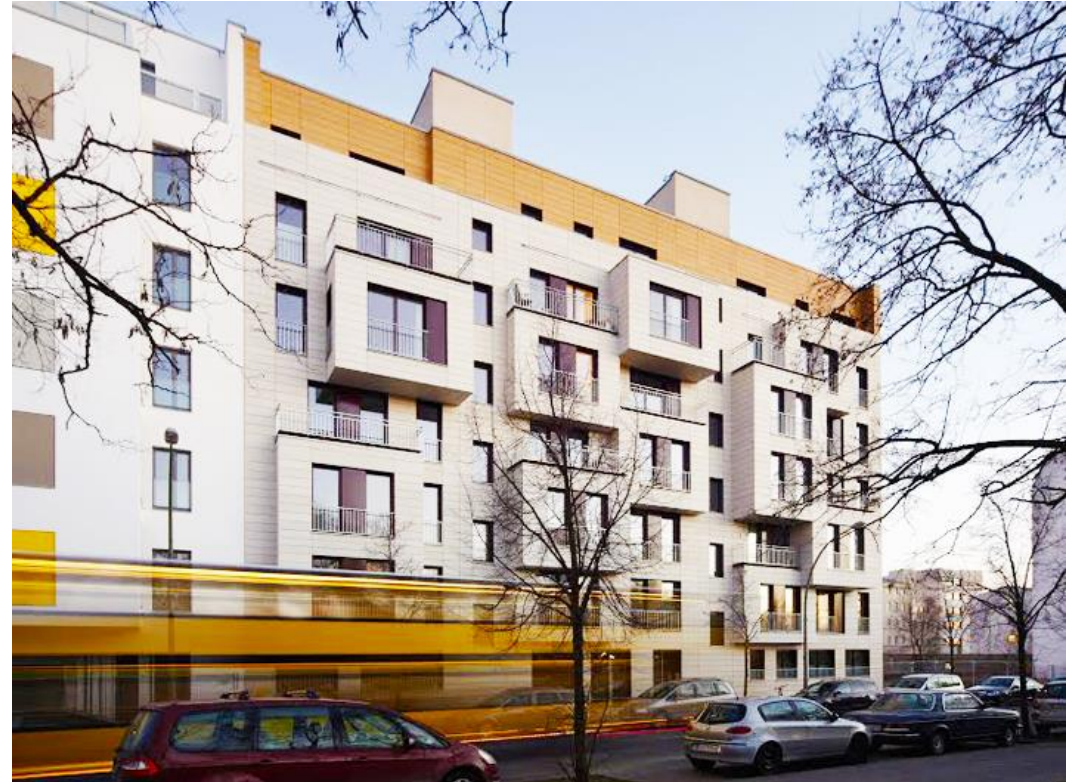
Zero emission apartment building Berlin, Germany
