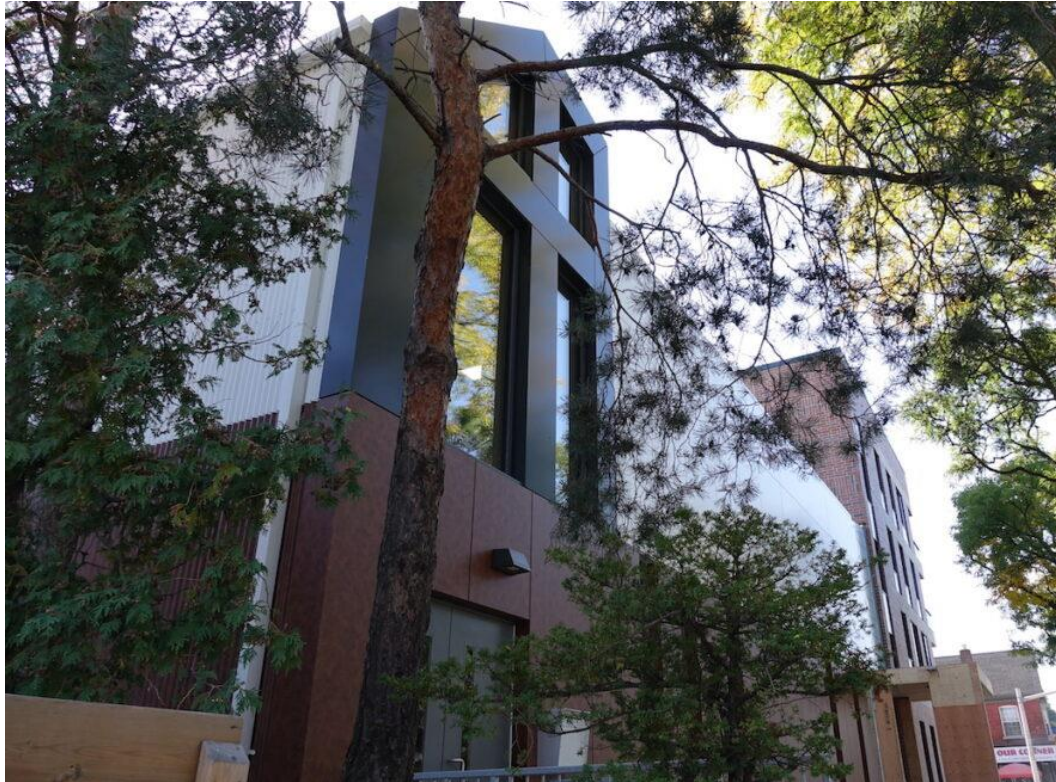
Passive House affordable housing development North End Landing Hamilton, ON
