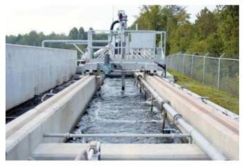
Figure 3-1 Grit Removal Channel
