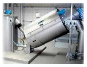
Figure 8-7 Rotary Screw Thickener (Courtesy of Huber)
