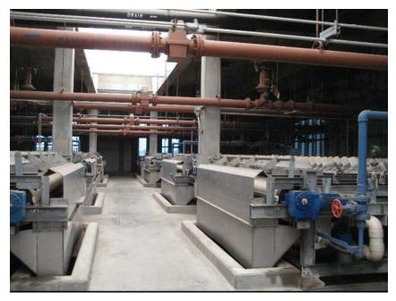
Figure 8-5 Installed Gravity Belt Thickeners at the Bissell WWTP
