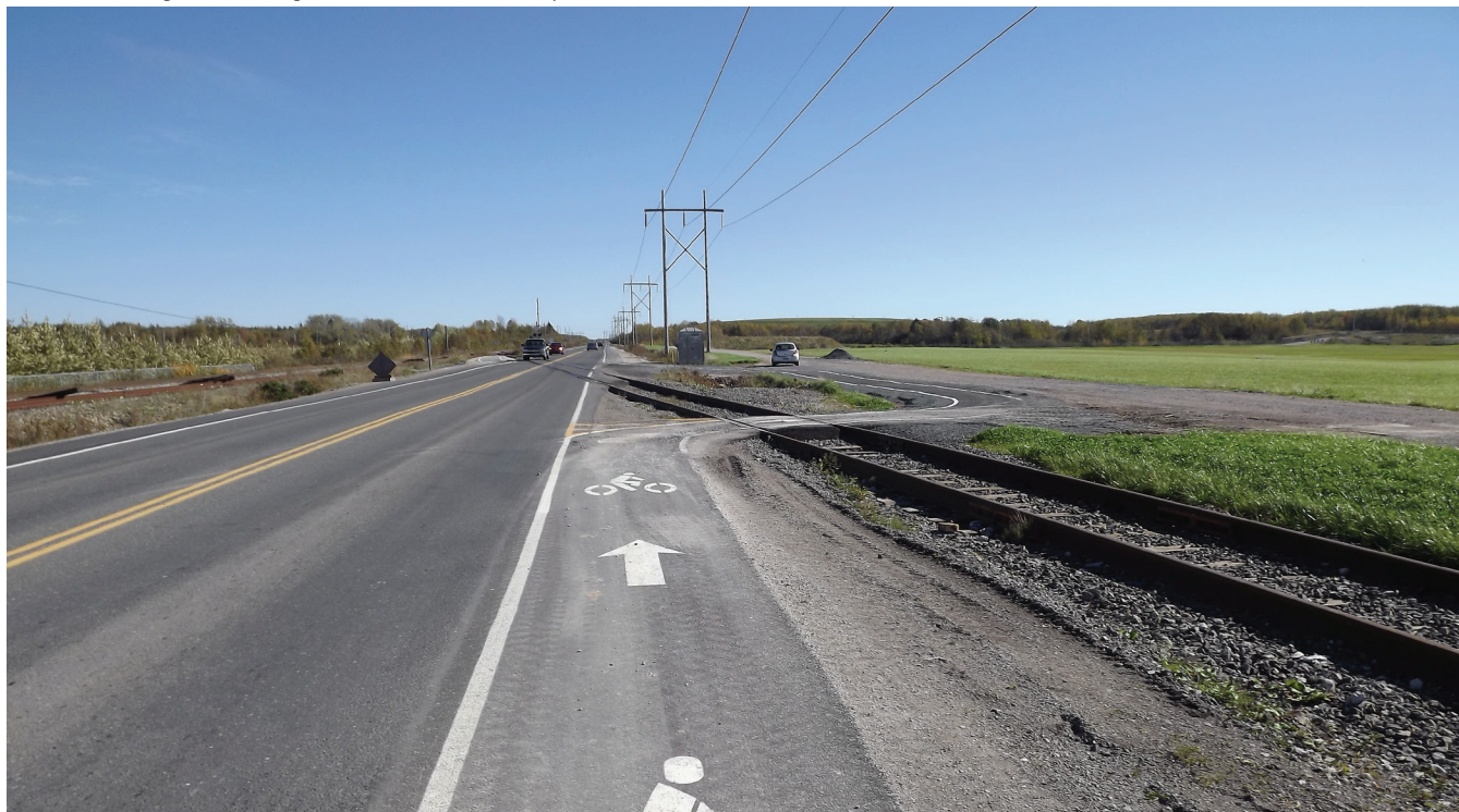
Exhibit 5-38. Jughandle Design for a Dedicated Bikeway with Sidewalk
