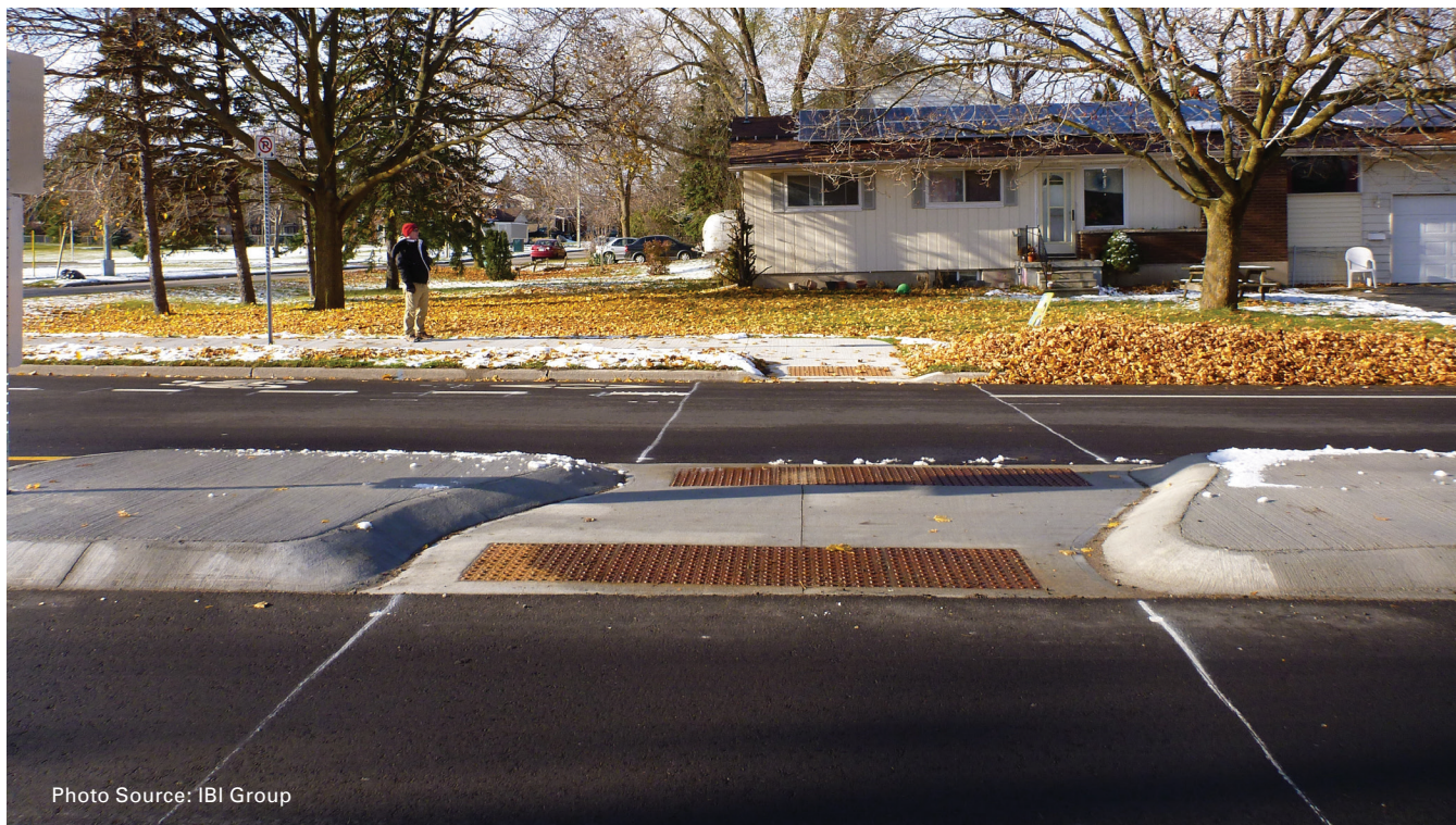
Exhibit 5-45. Use of detectable curbs to guide pedestrians through median refuge island
