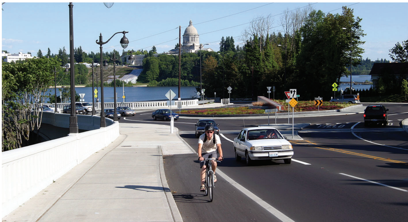
Exhibit 5-61. Example of a multi-lane roundabout with shared boulevard facilities through the roundabout
