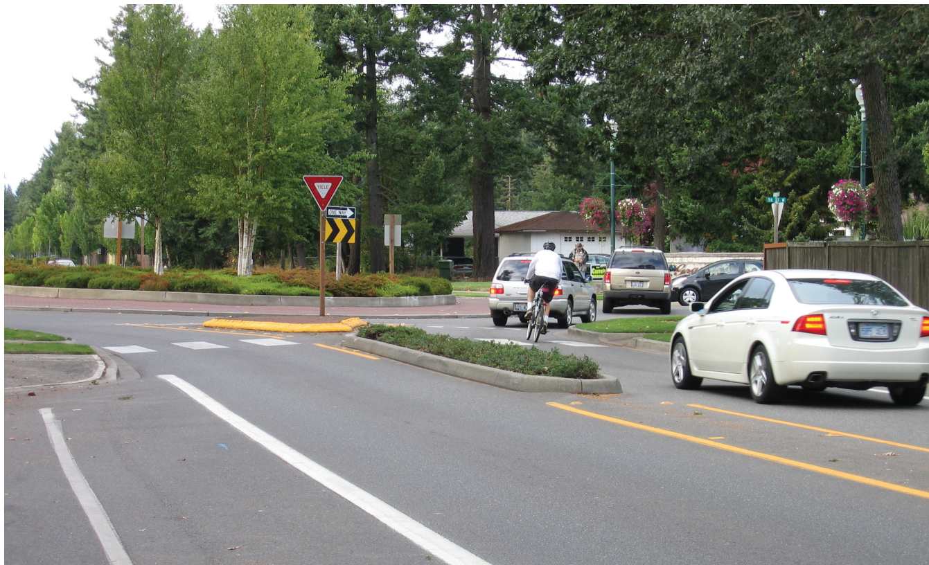
Exhibit 5-60. Example of a single lane roundabout with shared boulevard facilities through the roundabout
