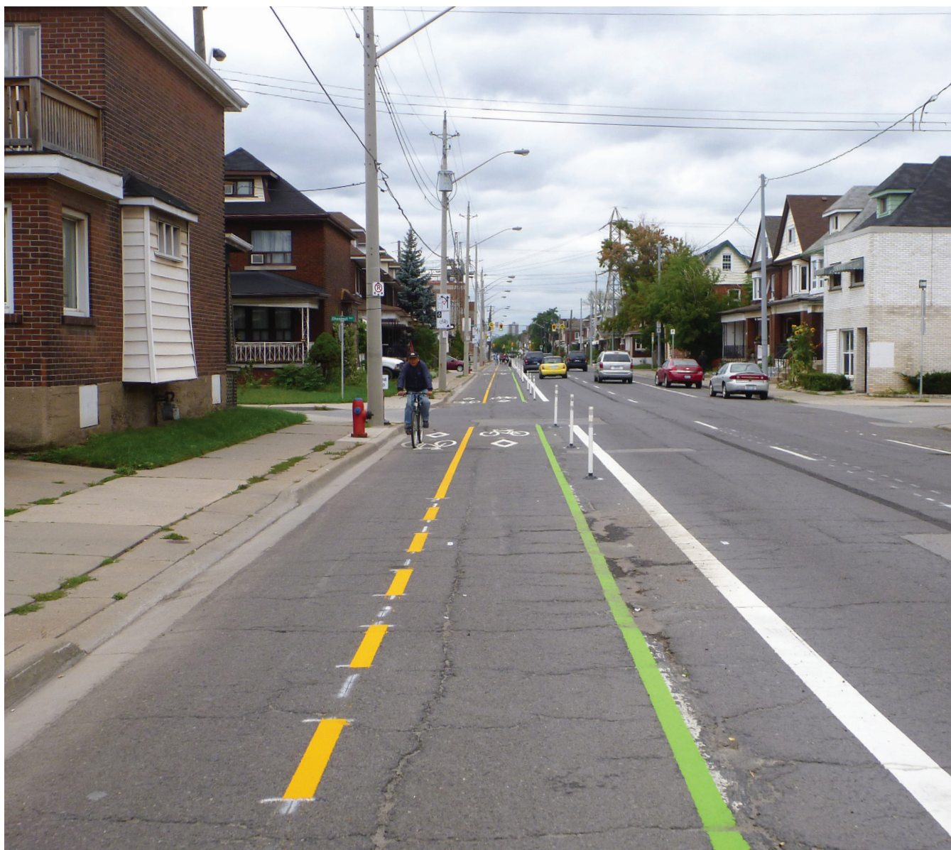
Exhibit 6-18. Solid buffer of separated bikeway carried across a multi-family residential driveway
