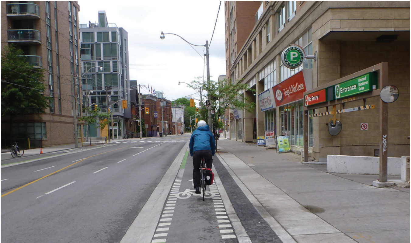
Exhibit 6-21. Example of high visibility treatments for cycle tracks at driveways
