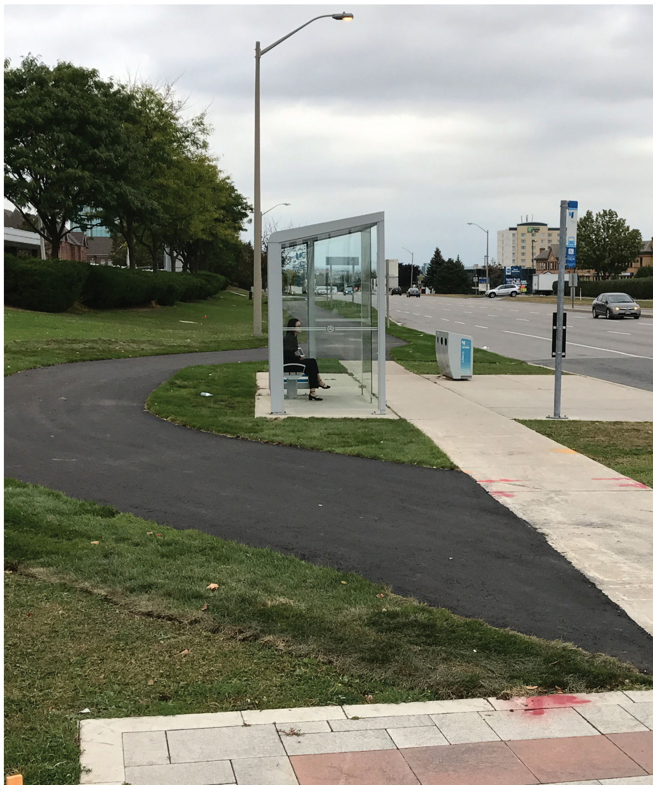
Exhibit 6-22. Example of a Multi-use Path bent behind a Transit Shelter in York Region
