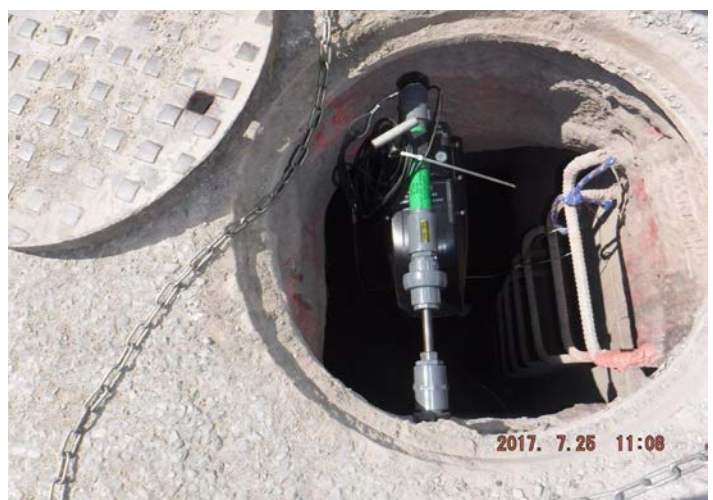
Figure 13: Level-only Flow Meter installed in the Town of Georgina
