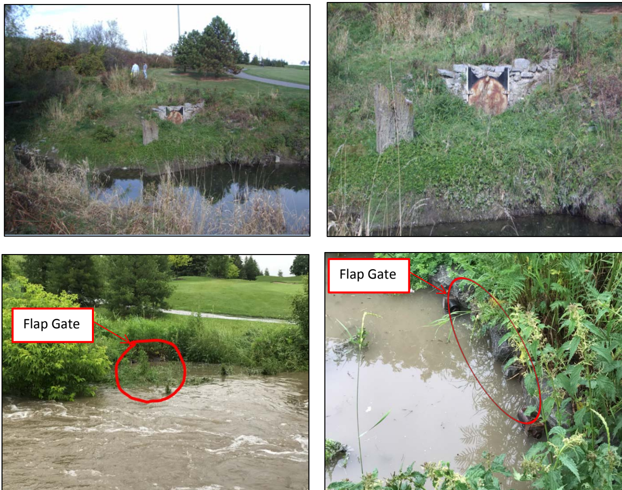
Figure 16 –Aurora Sewage Pumping Station Overflow Outfall Flap Gate location in comparison to the creek levels during dry and submerged conditions (During Jun 22-23, 2017 rainfall event)
