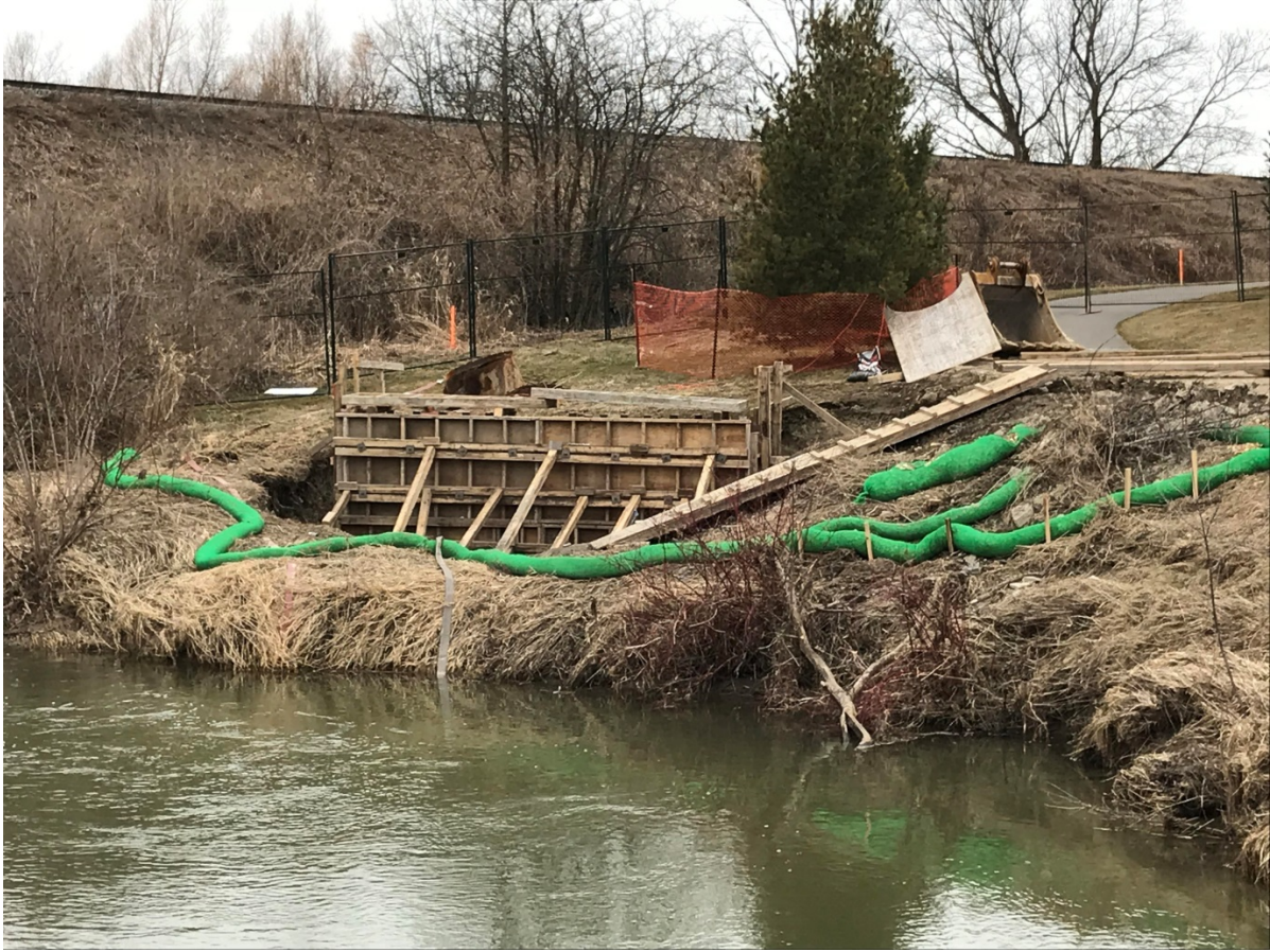
Figure B8 – Formation of the New Headwall
