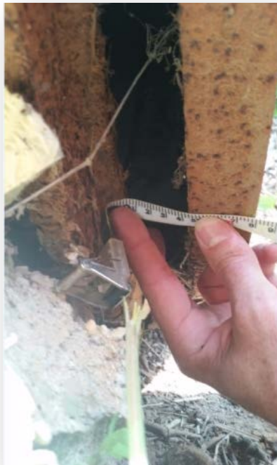
Figure 15 – Aurora Sewage Pumping Station Flap Gate Opening and Field Measurements
