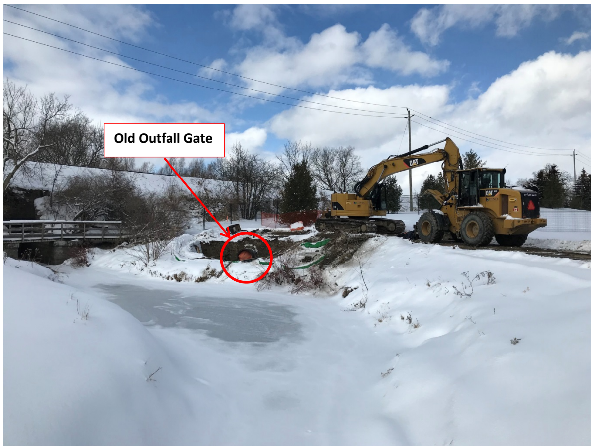
Figure B7 – Construction Zone after Removing the Old Headwall
