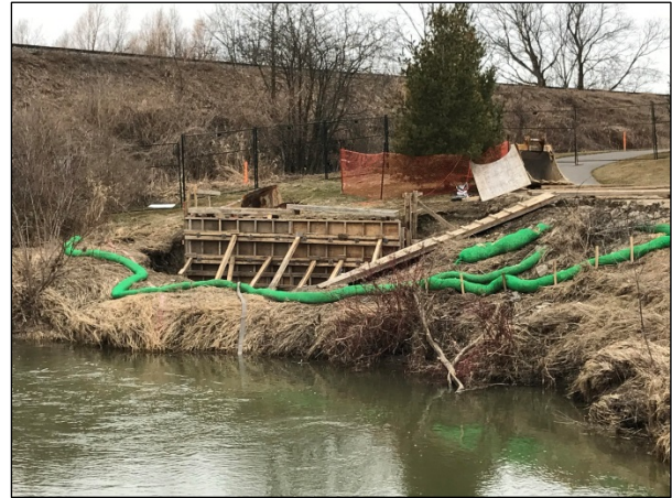
Figure 19 – Construction Zone after Removing the Old Headwall (Left) and Formation of the New Headwall (Right)
