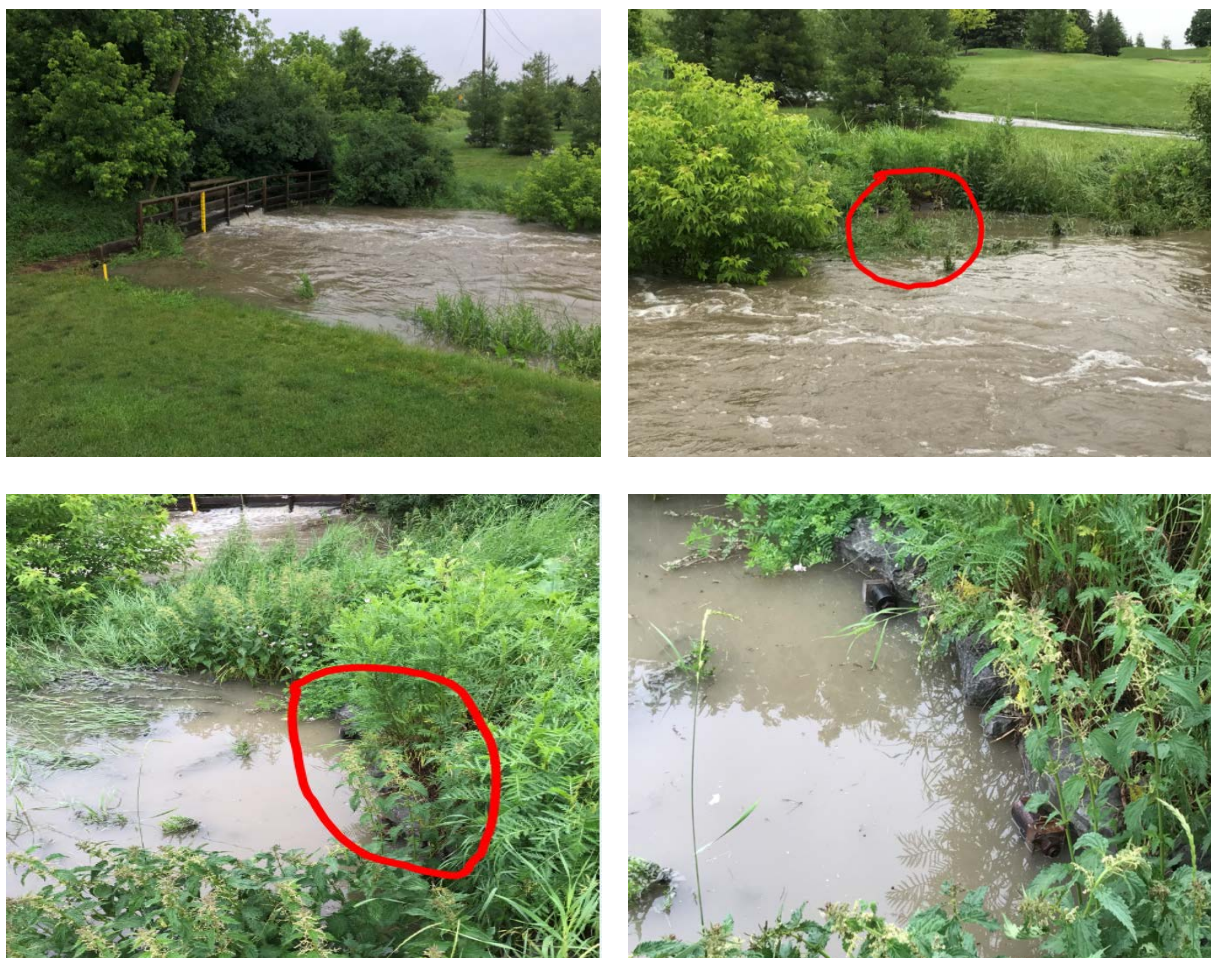
Figure B1 – Images of Submerged Condition of the Aurora Sewage Pumping Station Outfall Flap Gate – June 23, 2017
