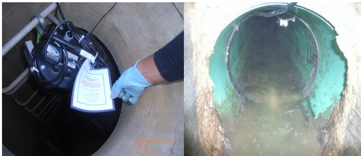
Figure 5: Pictures showing Area Velocity Meter and Sensor installed as part of the Flow Monitoring Program
