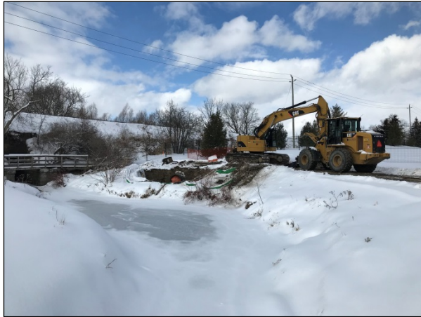
Figure 19 – Construction Zone after Removing the Old Headwall (Left) and Formation of the New Headwall (Right)
