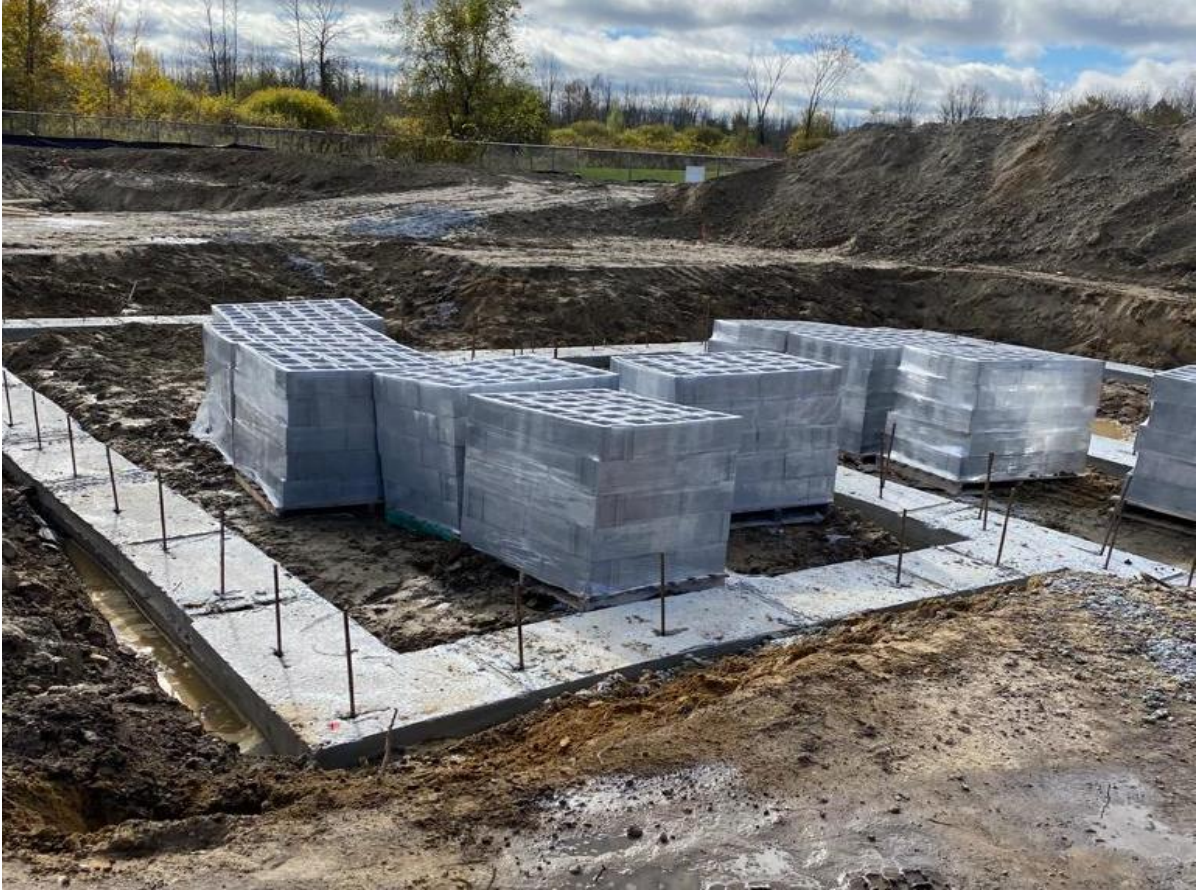
Building foundation and footings installation
