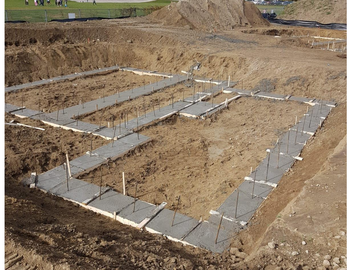
Pouring the building foundations
