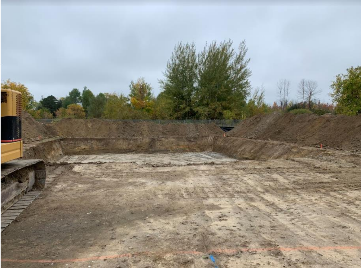
Excavating building foundations
