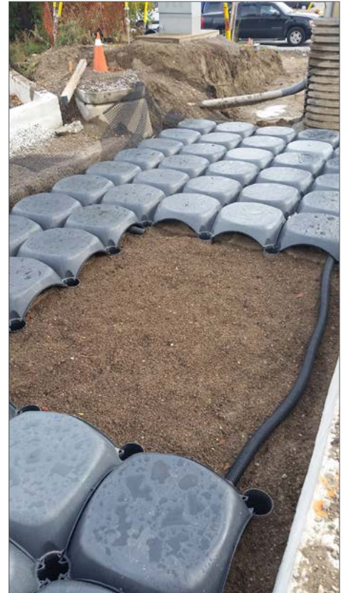
Installation of soil cell system within the boulevard.
