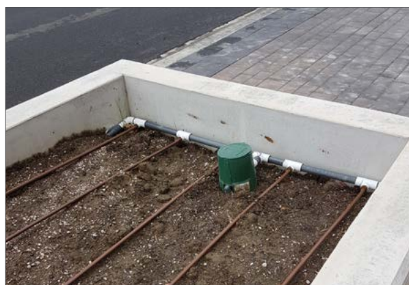
Example of dripline irrigation system being installed in a boulevard planter.
